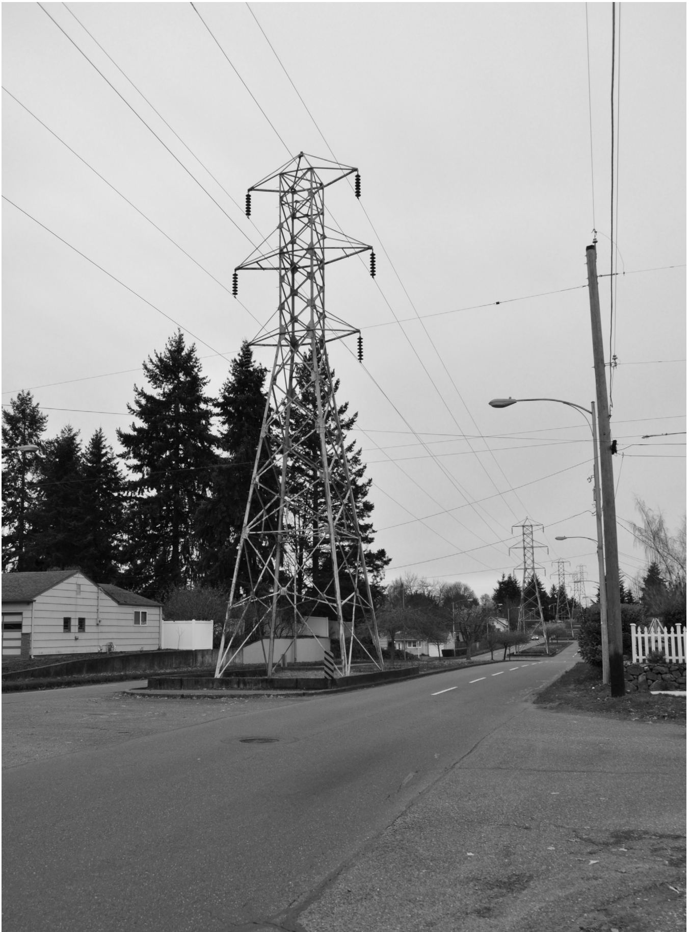
12 figure 4. high voltage transmission towers north 21st street
