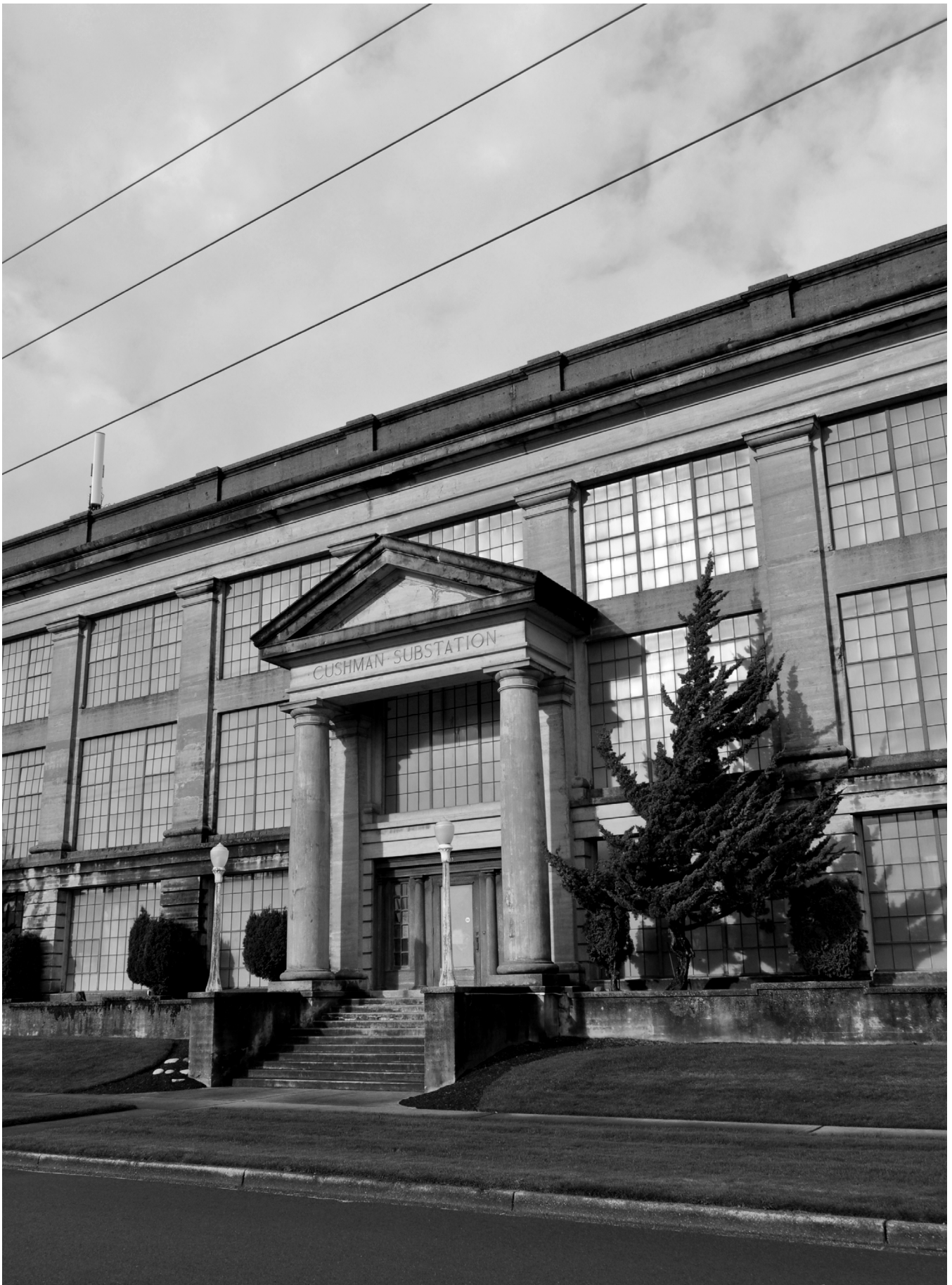
62 figure 44. the cushman substation main entry
