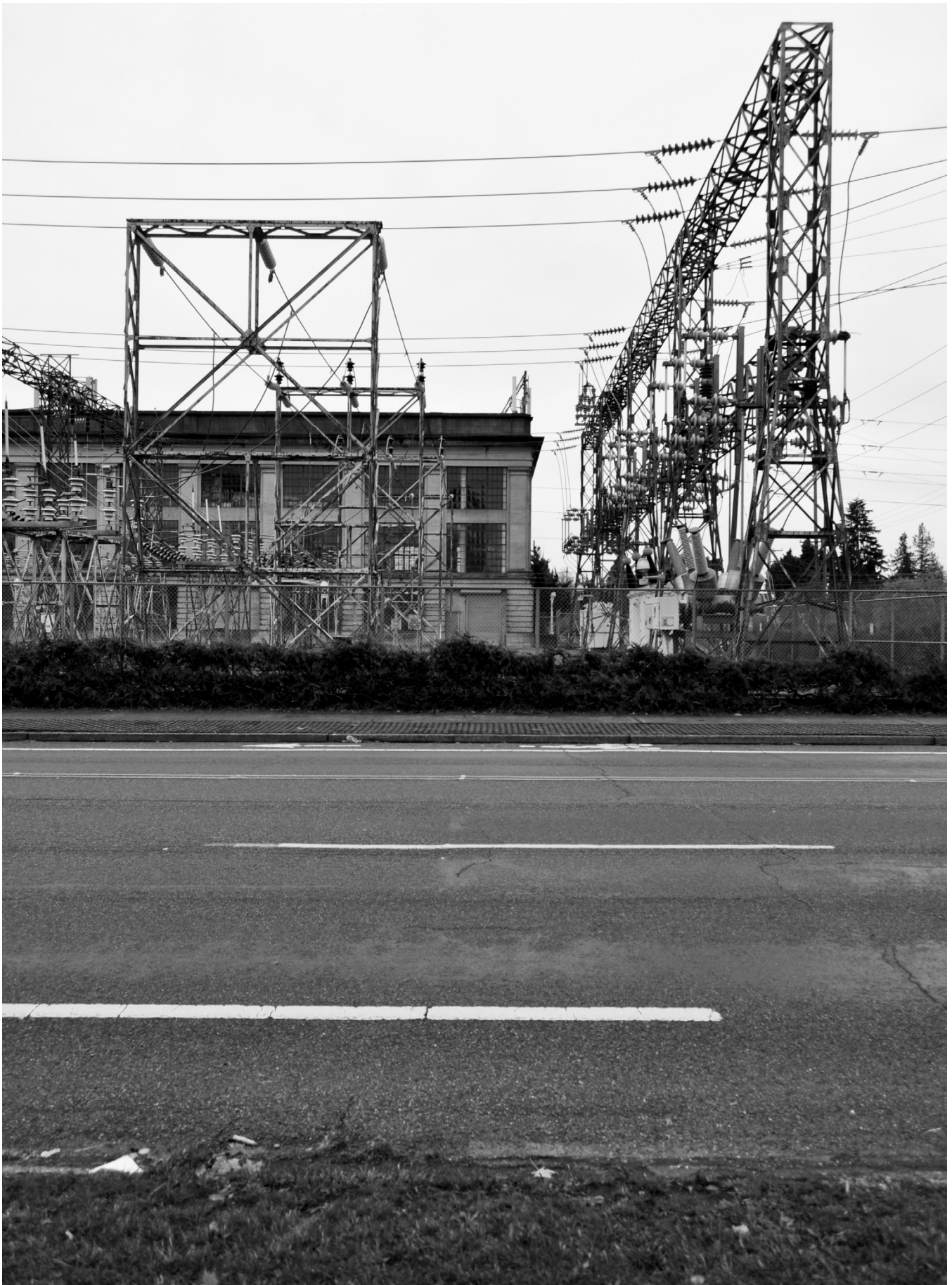
36 figure 25. existing infrastructure, lattice framework
