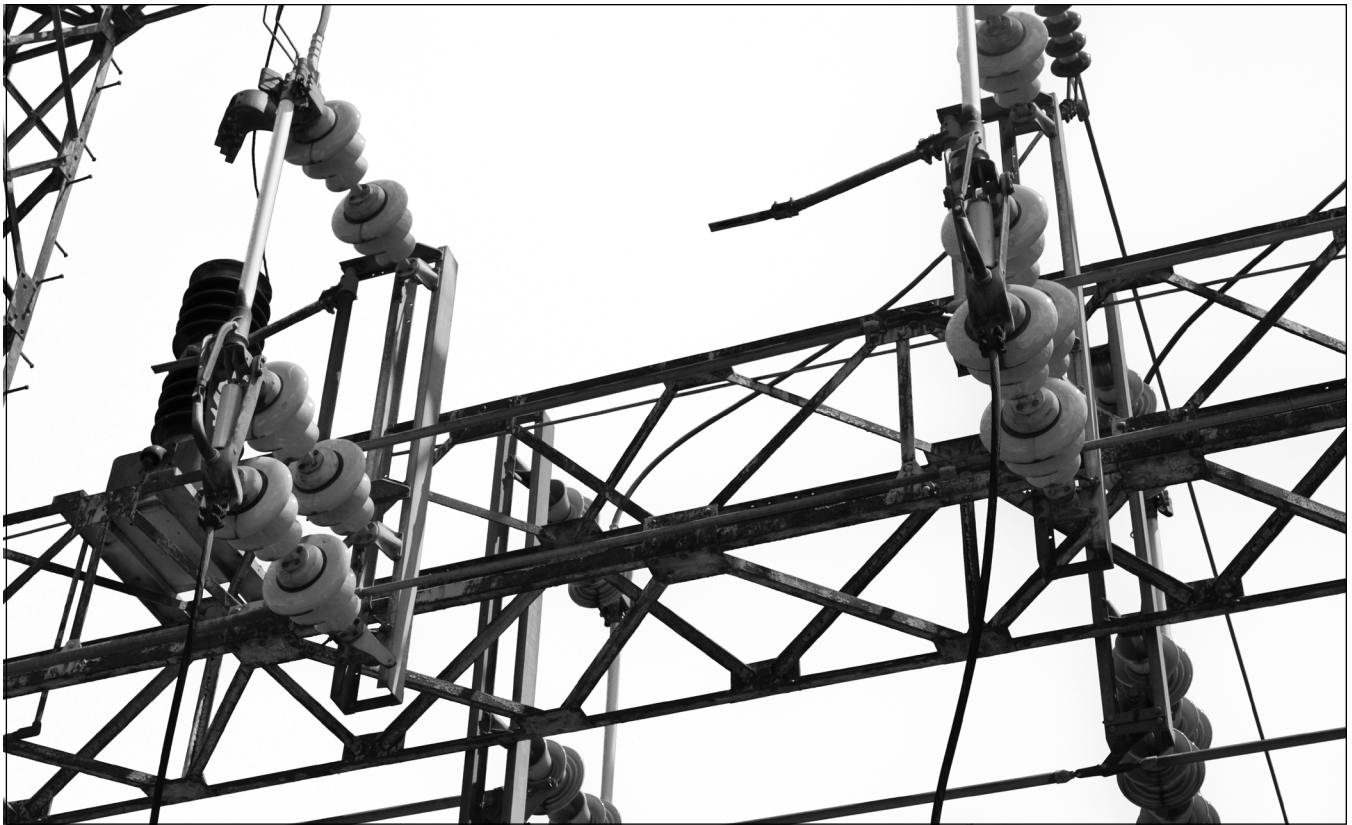
figure 29. existing steel lattice frames w/ original electrical components
