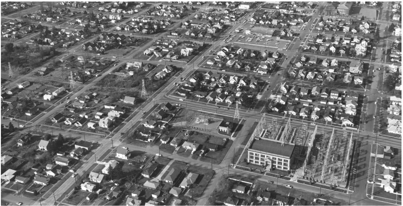
figure 15. southeast aerial view cushman substation and neighborhood, 1963
