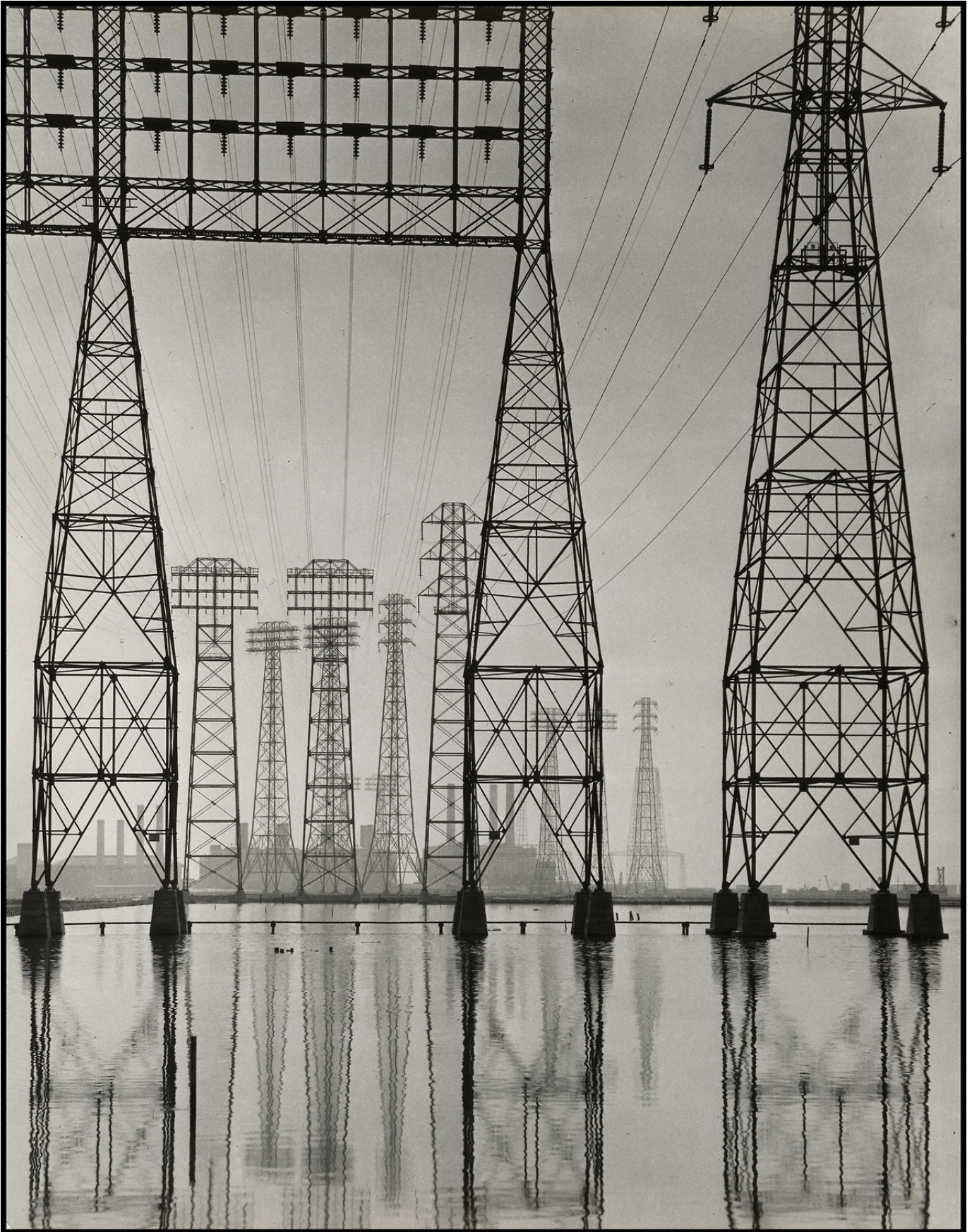
18 figure 7. pylons at seal beach, ca 1936, will connell
