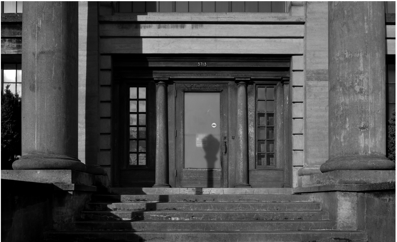
figure 3. cushman substation doric temple entry: "danger high voltage keep away"
