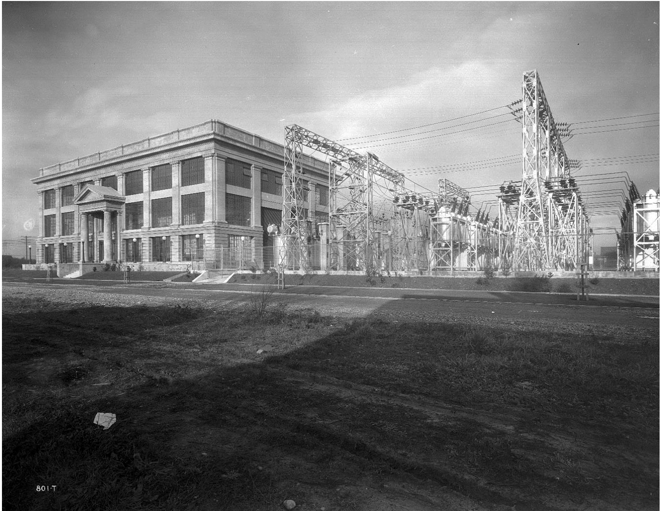
figure 27. cushman substation and switchyard 1926
