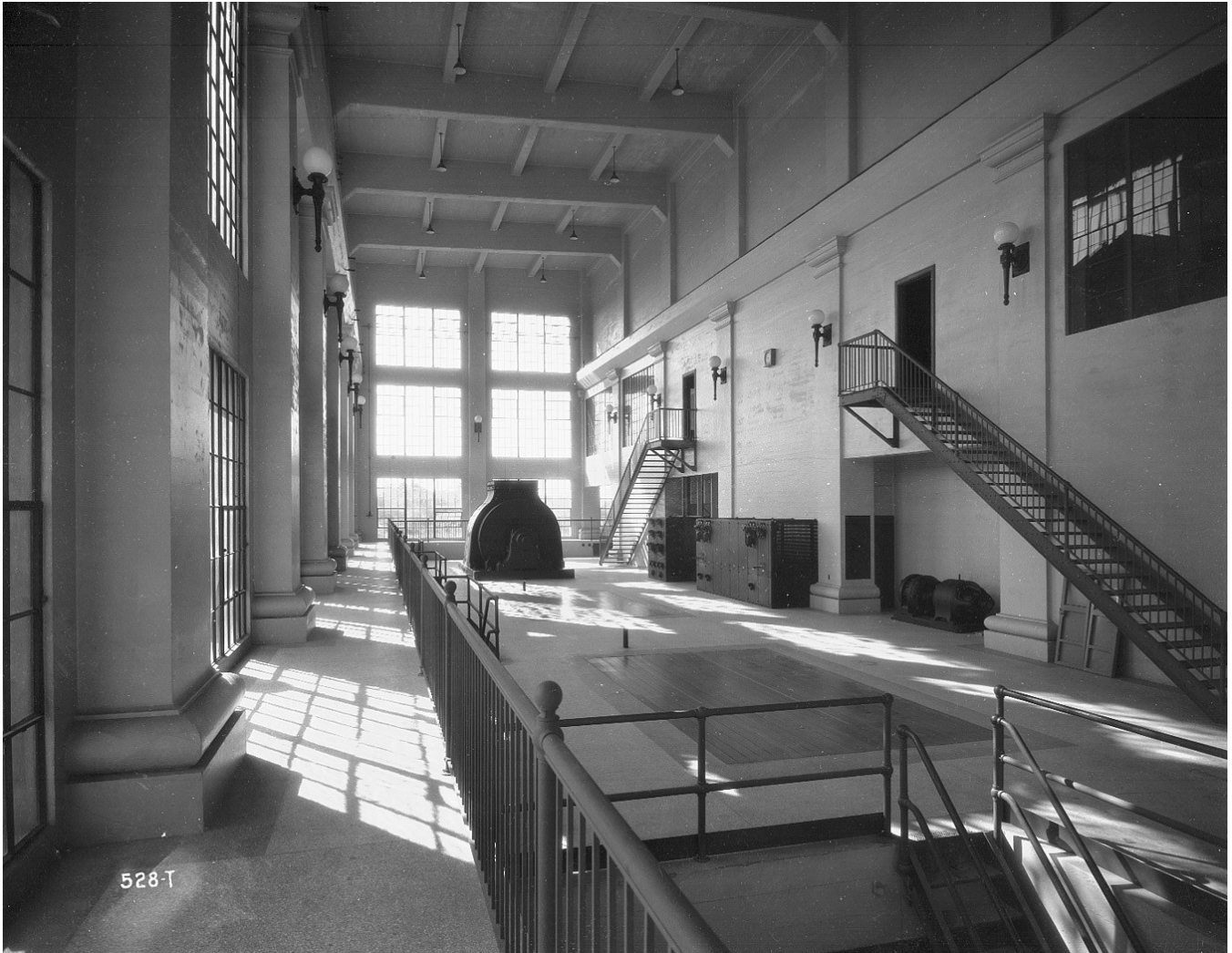
figure 28. cushman substation condenser room 1926
