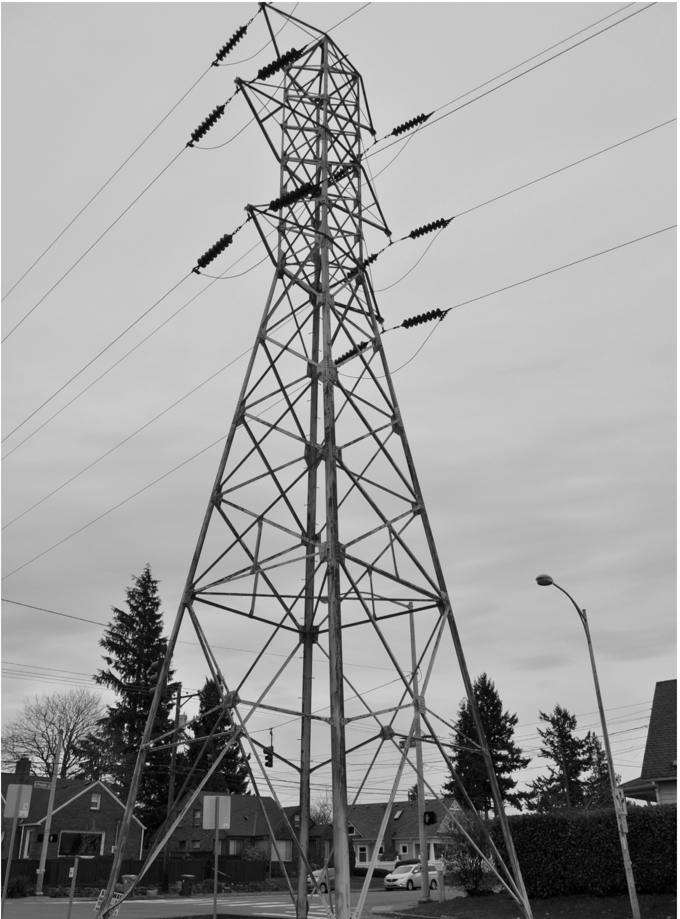
34 figure 24. high voltage transmission tower
