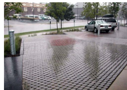
Figure 5 Permeable Pavement Source: http://nacto.org/
