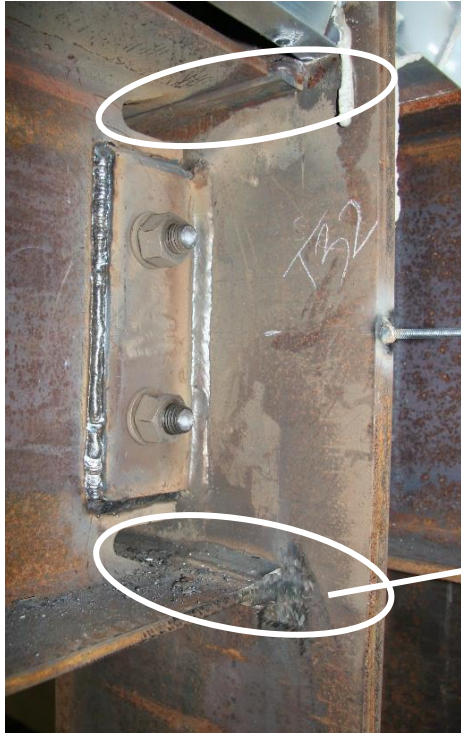
(a) backing bars on welded connection
