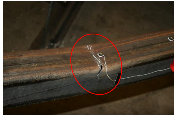
Figure 4.29 S brace @ 3.3% drift
