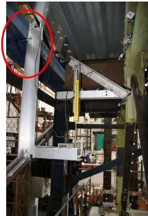
(a) Second Story beam
