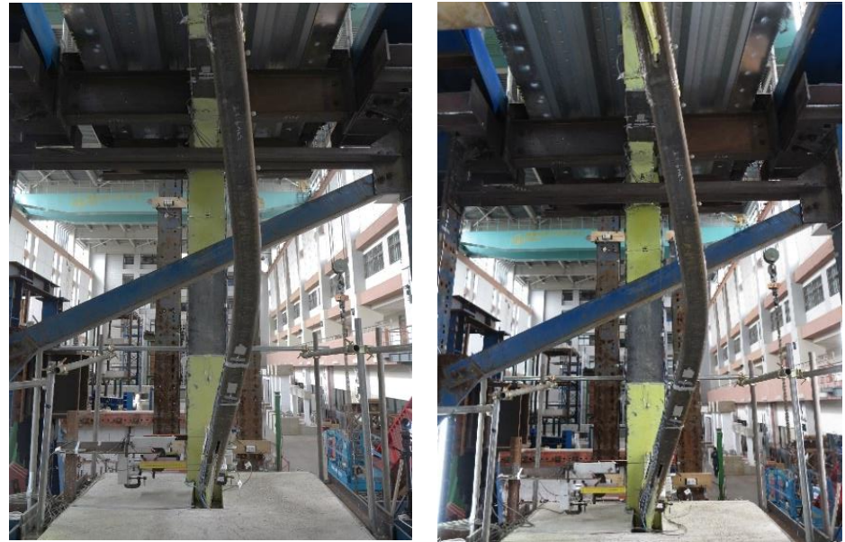
(a) 0.9% roof drift
