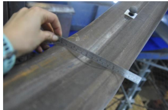
(b) 2SBr at -3% roof drift
