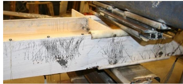
(a) Chevron 3 beam yielding
