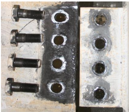
Figure 4.52 Final Condition North Beam Web and Shear Tab
