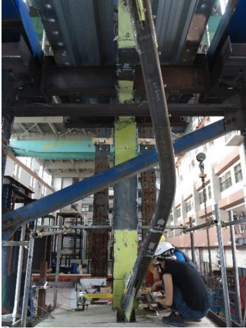
(c) 2NBr 1.8% roof drift
