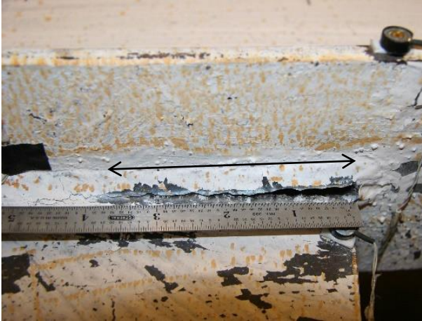
Figure 4.24 N mid gusset weld crack @ 2.8% drift
