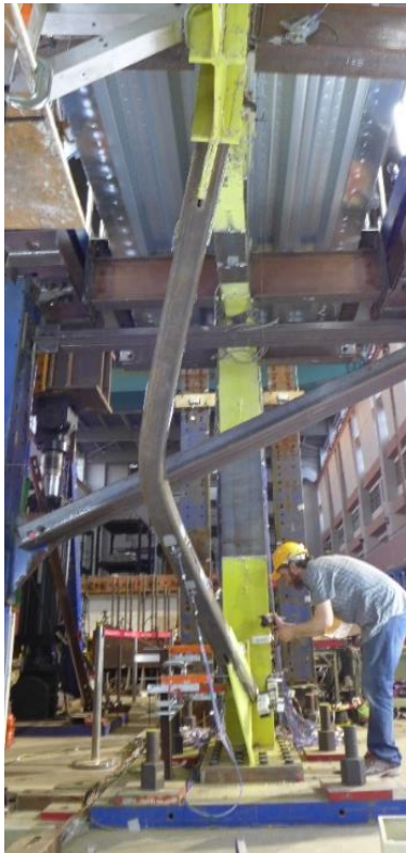
(a) 1NBr 1.8% roof drift
