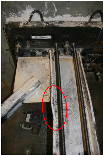
Figure 4.50 Local yielding/buckling at S Column base 3.65%
