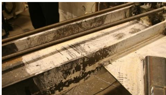
(b) Chevron 1 north column
