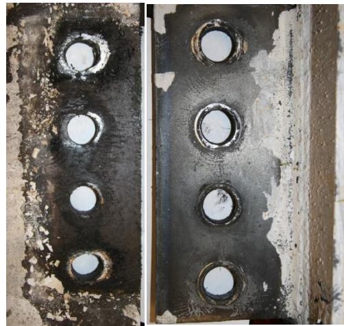
Figure 4.70 Final Condition North Beam Web and Shear Tab
