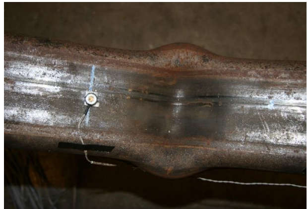
Figure 4.66 S brace @ first cycle -3.0% drift
