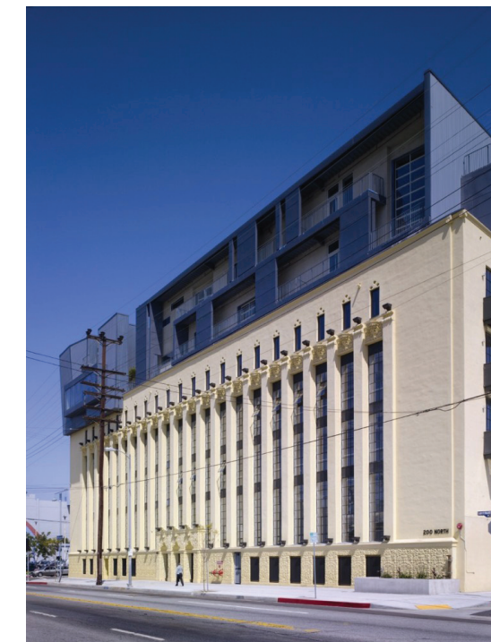
Figure 4.13: Before and after images of the Fuller Lofts. Images from Pugh + Scarpa.
