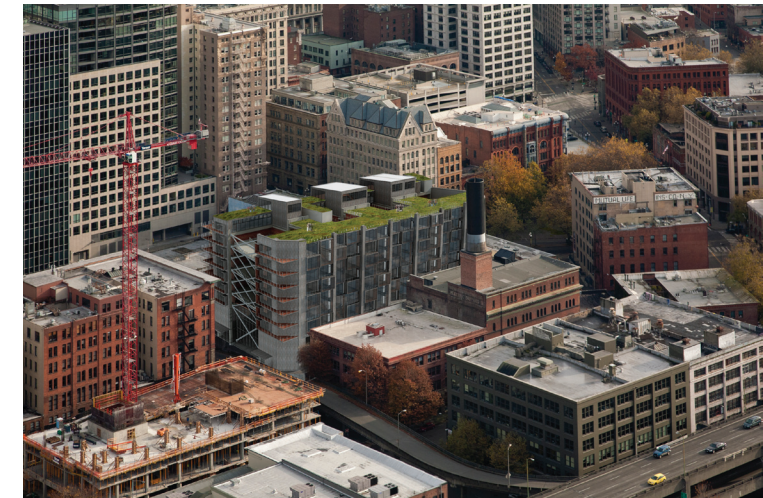
Figure 6.23: Bird's eye view of the building and surrounding context before and after reuse.
