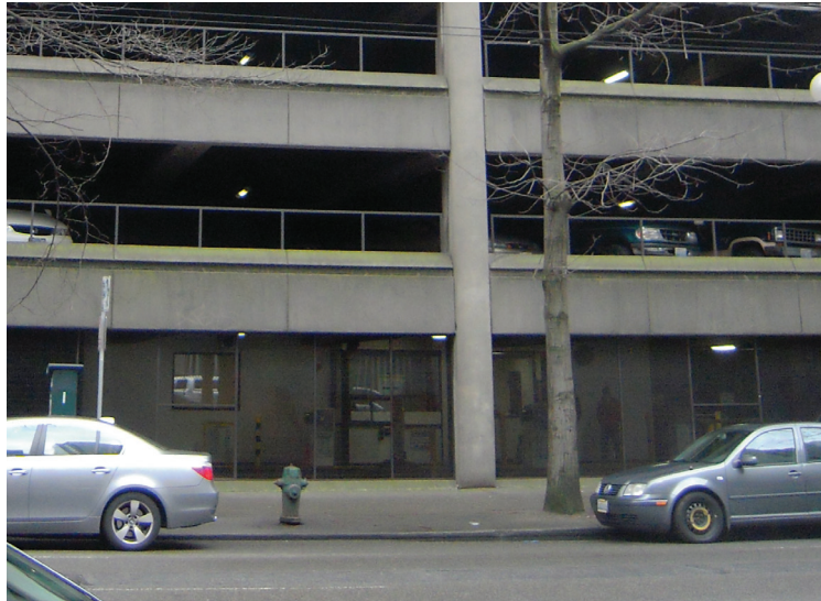
Figure 2.8: The face of the existing column sits at the property line of many garages, such as this one.
