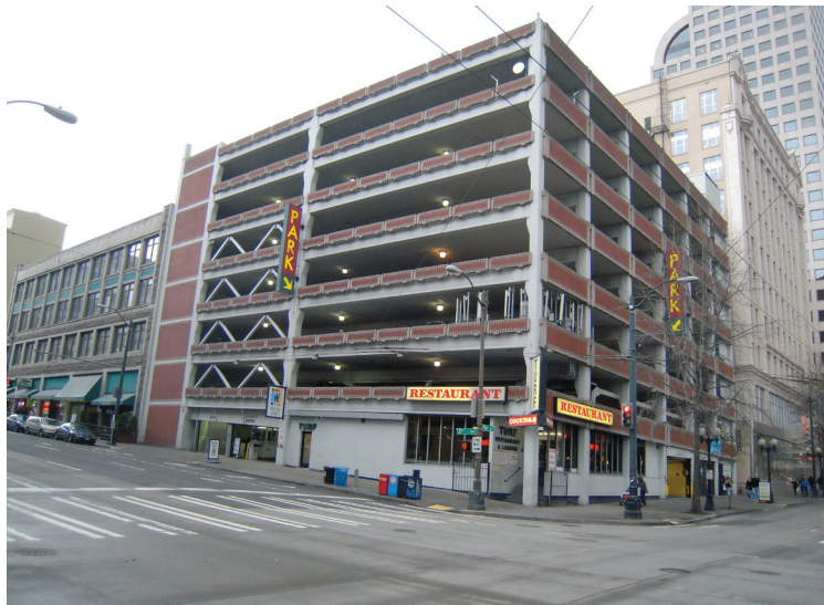
Figure 2.9: Concrete panels with inlaid brick are attached outside the line of structure. Removing them would provide some space between the existing structure and the property line.
