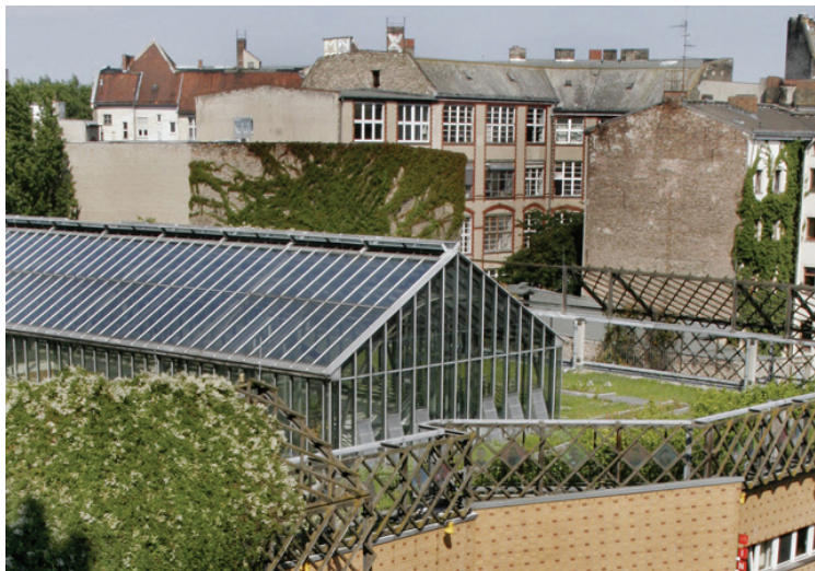
Figure 4.4: Rooftop green house and open space
