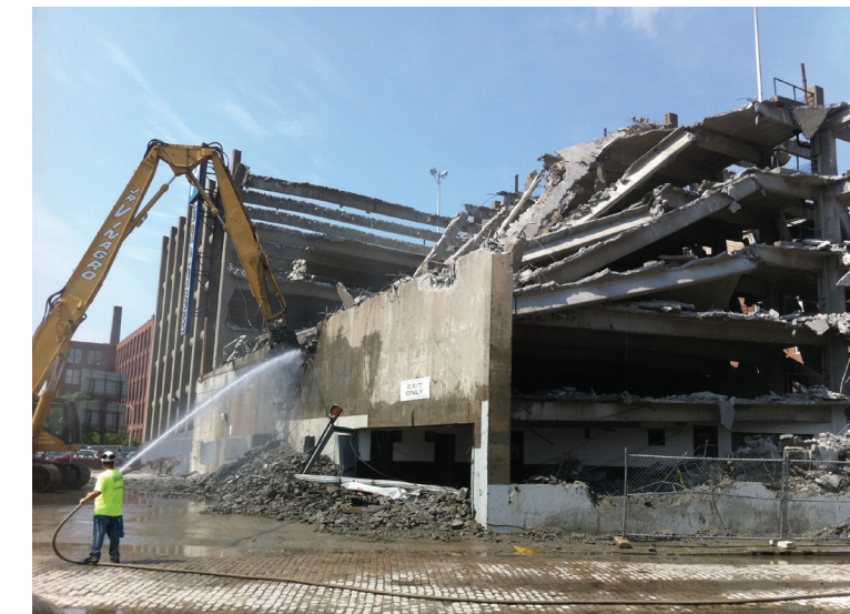
Figure 3.1: Concrete parking garages undergoing demolition.
