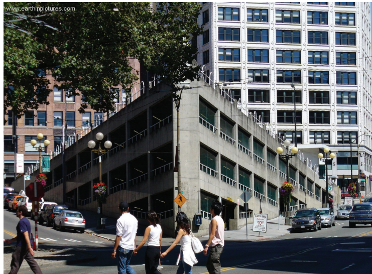
Figure 2.5: The Triangle parking garage in Seattle's Pioneer Square has four sloped levels that act as both circulation and car storage
