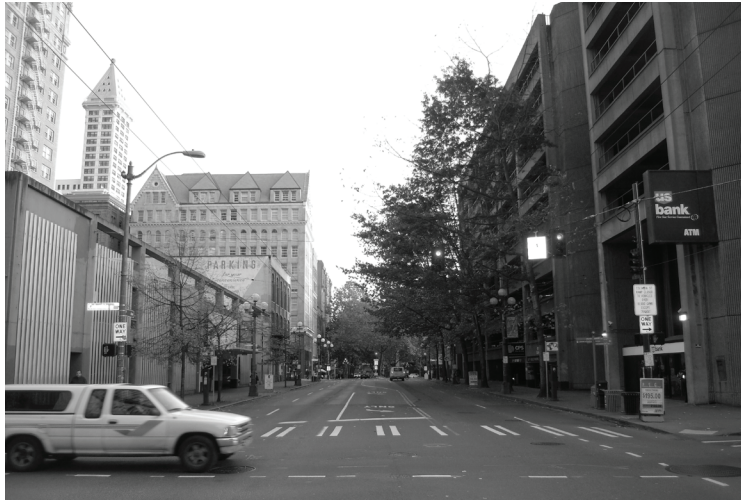
Figure 5.6: 1st Avenue between Columbia Street and Cherry Street. Parking garages currently form the street wall of the entire 250 foot long block.
