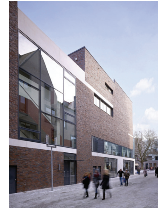
Figure 4.11: The existing brick facade was deconstructed in places and curtain walls were added to bring in light. Photo credit G. Erbring
