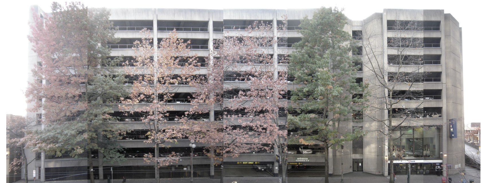
Figure 5.7: 1st Avenue elevation of the garage at 701 1st Avenue.
