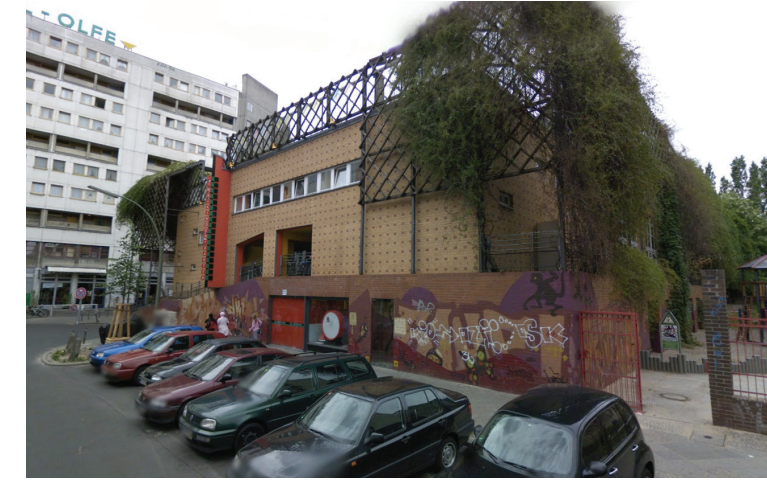
Figure 4.5: Street view of reused garage highlighting steel lattice structure supporting vegetation.
