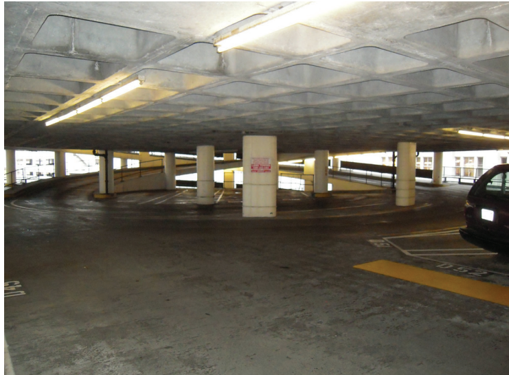
Figure 2.4: Double spiral ramp in the Bon Marche garage
