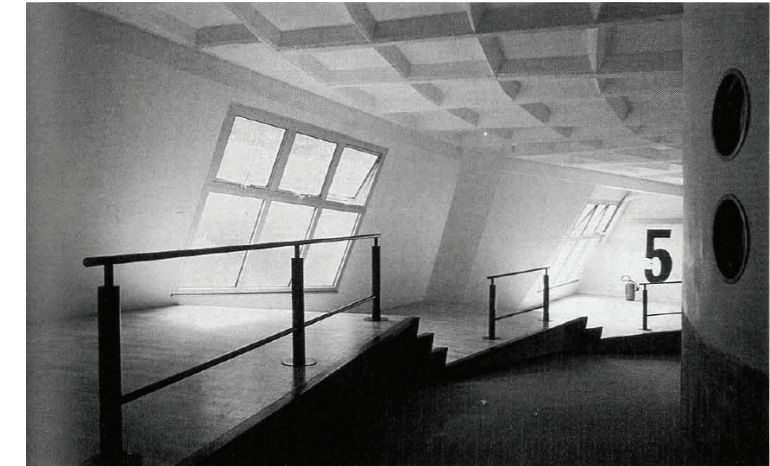
Figure 2.6: Existing parking ramp with insertion of new stepped platforms to create usable space on the sloped surface. Office of Liberation Newspaper, Paris, France. Photo from Architectural Record
