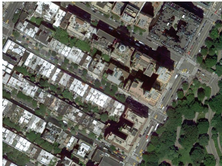
Figure 6.11: Aerial view of buildings with light courts along Central Park West.
