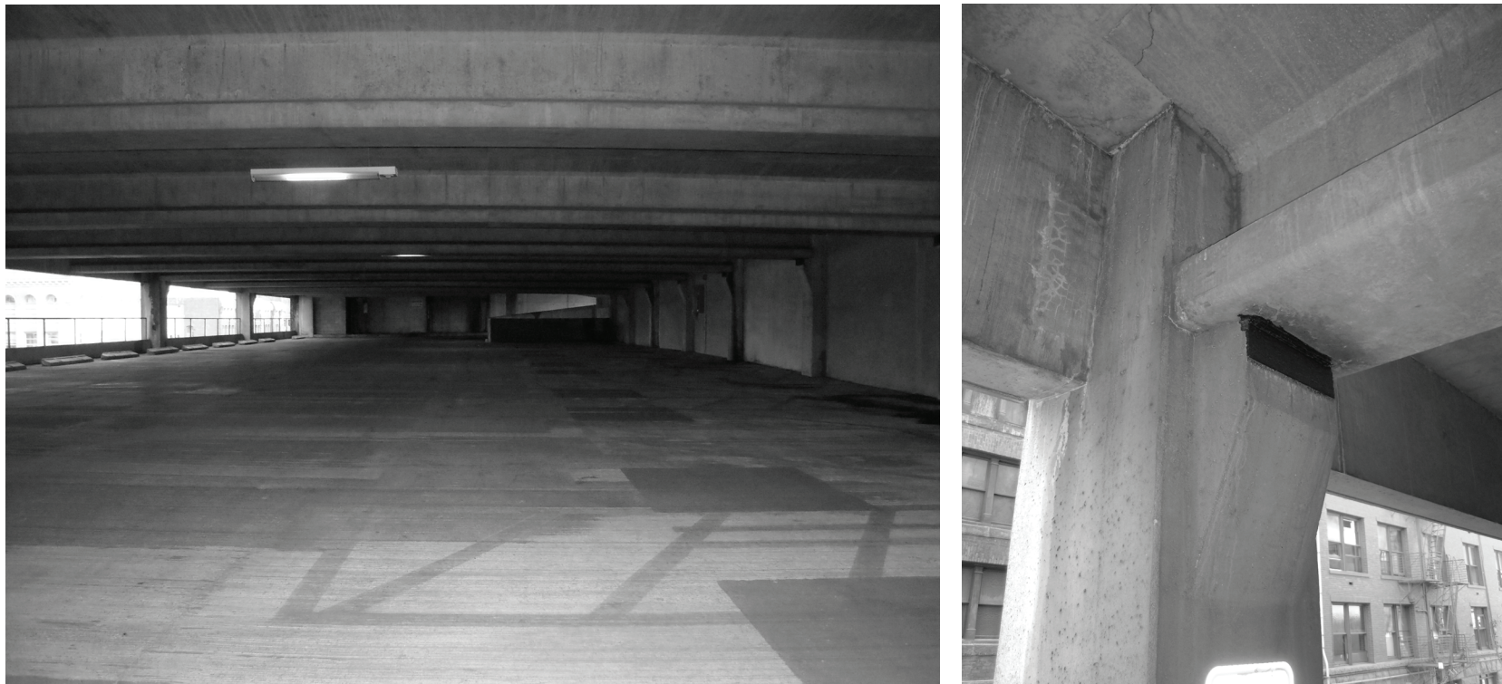
Figure 6.1: Photographs depicting interior conditions of the existing garage.
