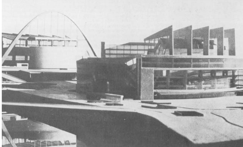
Figure 3.9 – Roof suspended by tension cables, hung from parabolic arch in Le Corbusier & Jeanneret, Palace of Soviets Project, 1934. (Le Corbusier, Pierre Jeanneret, Willy Boesiger, Oscar Stonorov, and Max Bill, Oeuvre complete: Volume 1 . (Zürich: H. Girsberger, 1935), 130.)
