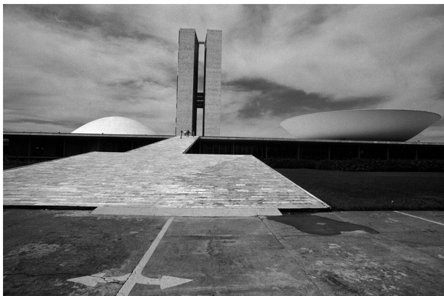
Figure 4.25 - Le Corbusier's Chandigarh Assembly Hall (1952, top) and Oscar Niemeyer's Brasilia Assembly Hall (1956, bottom). (Top Image: Cities and Buildings Database, Copyright
