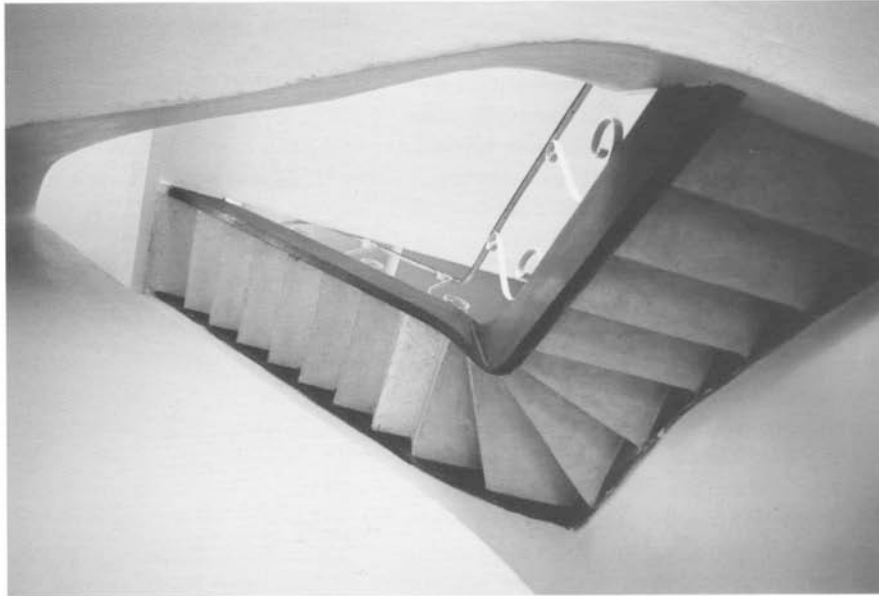
14. The house belonging to M. Nowicki's parents in Warsaw, inner staircase.
