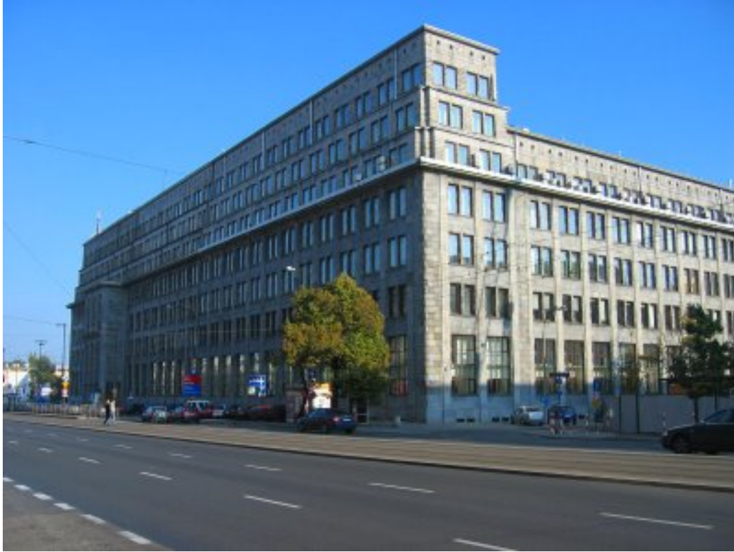
Figure 2.2 - Swierczynski's Ministry of Transport Building, ca. 1928-31. (Image source: Mike Roman, http://wandersthroughwarsaw.blogspot.com/2008/07/fifteen-per-cent-following-photographs.html )
