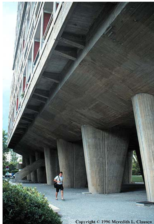
Figure 5.6 - Le Corbusier’s Unite’ d’Habitation, piloti, 1947. (Cities and Buildings Database, copyright Meredith Clausen, slide no. 2209, University of Washington)
