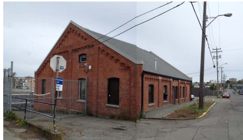
Figure 30: Photo of the current Victoria Gas Co. brick building
