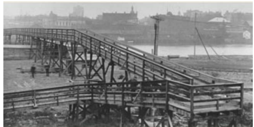
Figure 21: Pre-1900 Rock Bay Bridge
