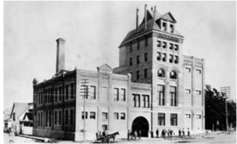
Figure 25: Victoria Brewing Company Building, designed by John Teague, built in 1892, was adjacent to the powerhouse
