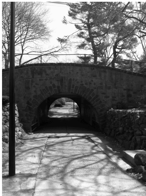
Image 1.5. Pedestrian underpass, vehicular overpass (both photographs taken by the author, April 11, 2014)
