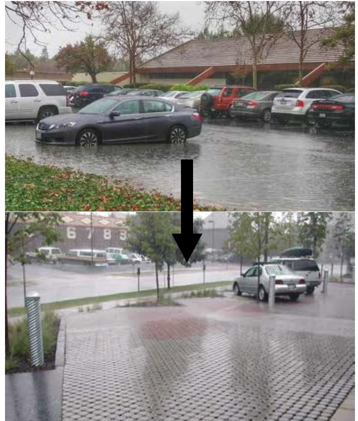
Figure 4.2.35 Permeable Paving at Work; (Source: ABC7 News; National Association of Transportation Officials)
