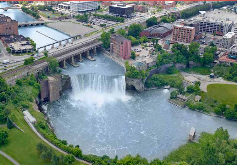
Figure 2.3.30 Aerial Photograph High Falls Waterfall (Source: City of Rochester, NY)
