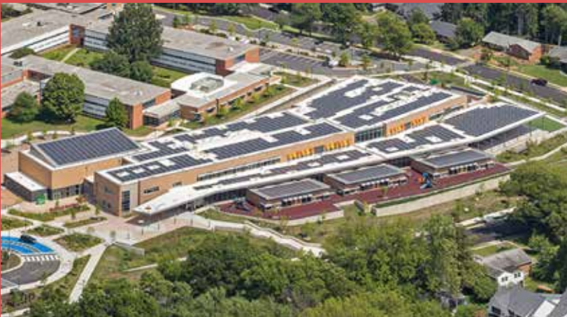
Figure 2.3.14 Roof-Top Solar Panels (Source: VMDO Architects)
