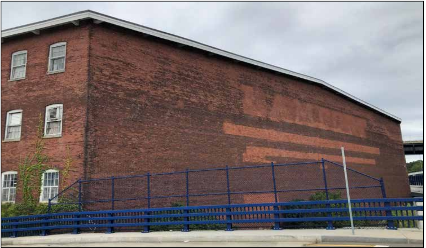
Figure 5.1.5 View of 104 Anawan East Facade (Source: Morgan Warner)
