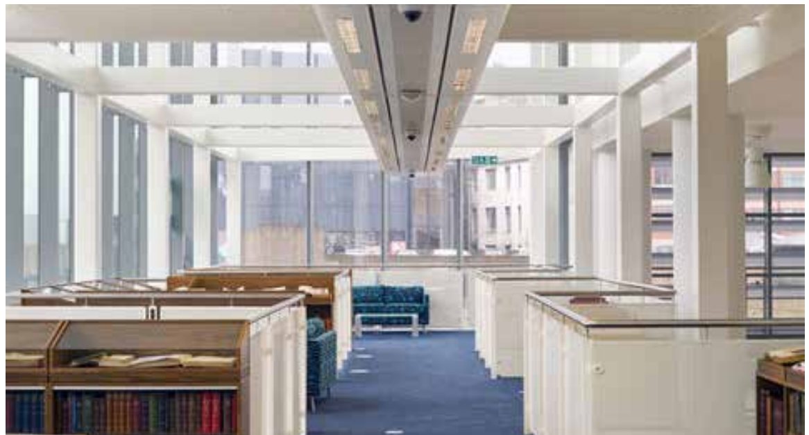
Figure 5.2.10 Chilled Beam; (Source: Building Green)
