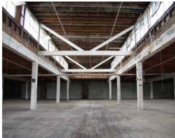
Figure 2.3.39 Building Condition Before Renovation (Source: Rice Fergus Miller)
