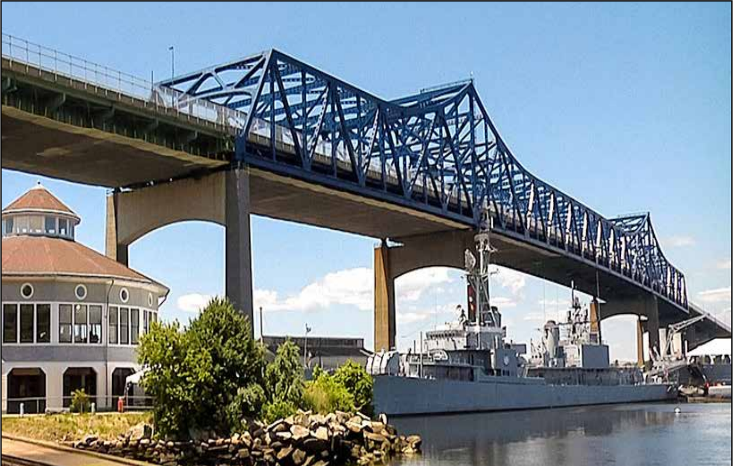
Figure 4.1.1 Night View of Braga Bridge (Source: Nancy Marshall)
