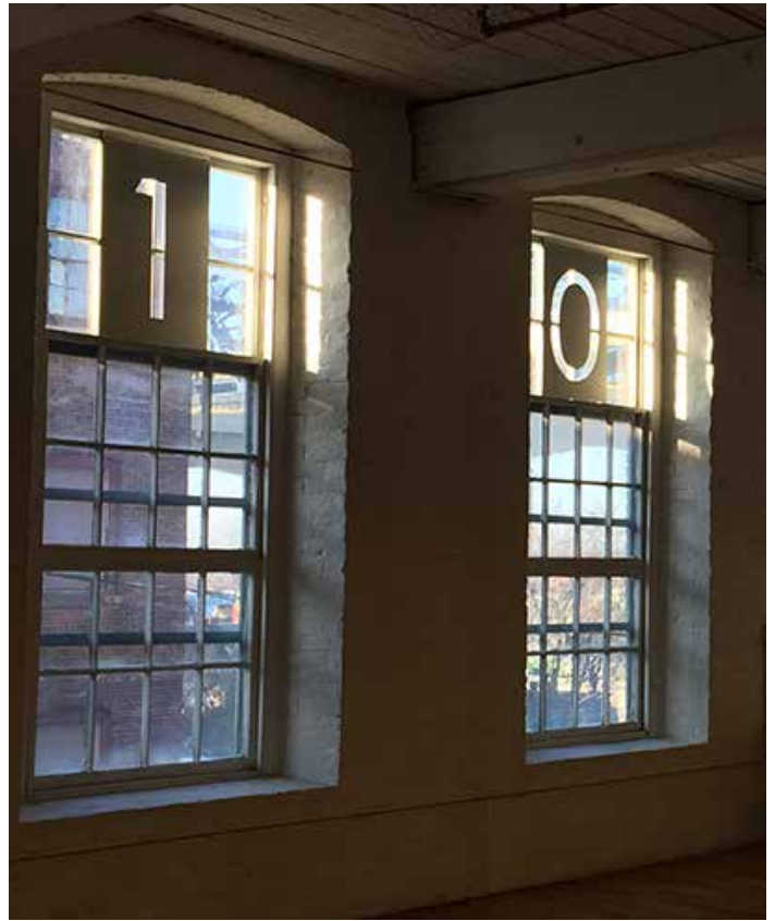
Figure 5.1.10 104 Interior Window Condition (Source: Morgan Warner)
