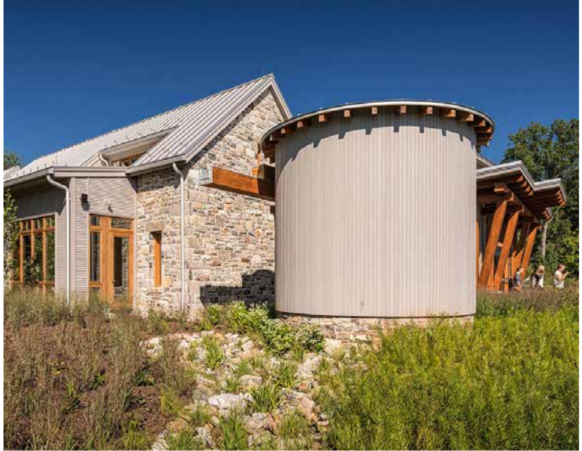
Figure 2.3.15 Water-Storage Cistern (Source: Farewell Architects)
