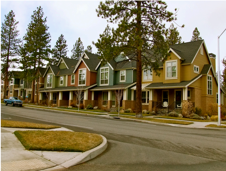
Multifamily Attached Housing in Northwest Crossing
