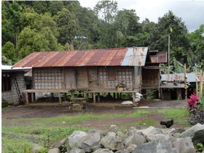
Figure 8.4: Village Residence, Takatunga Village
