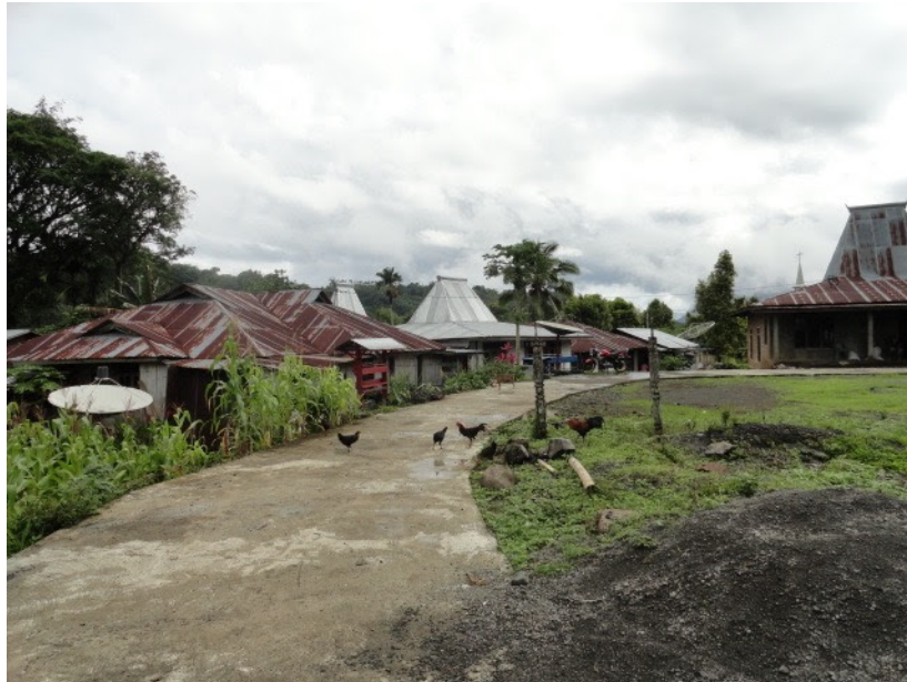
Figure 8.5: Concrete Road, Dariwali Village
