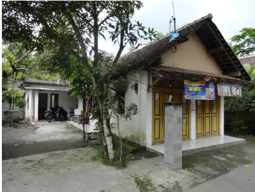
Figure 7.5: Village Residence and Shop, Baleharjo Village
