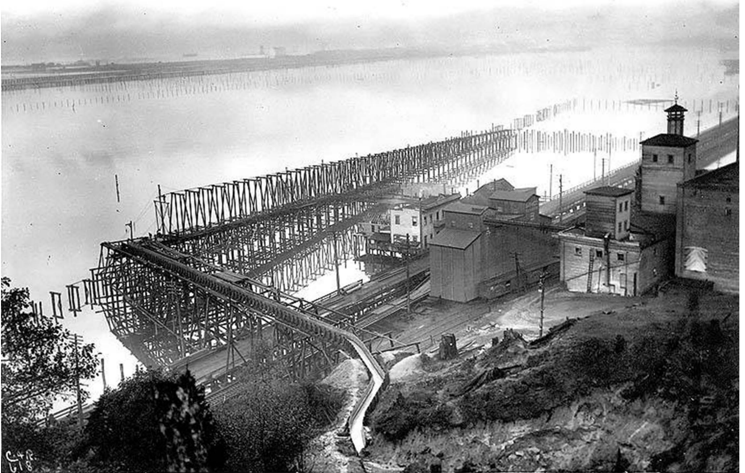
Figure 20. South Canal trestle; filling tideflats near Bay View Brewery, Seattle, 1901
