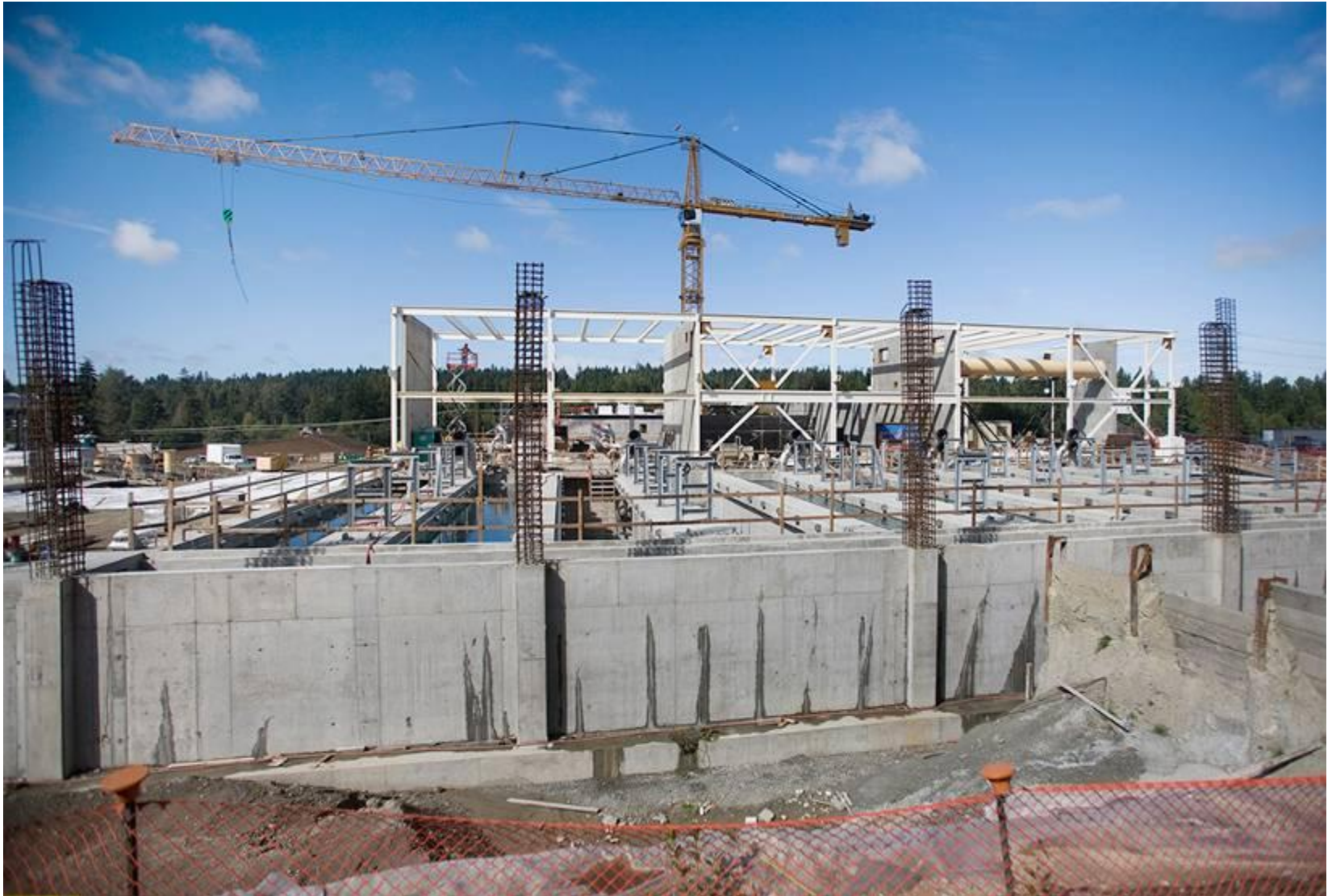
Outside wall of membrane building
