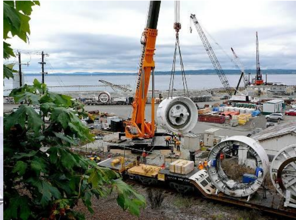
TBM delivery to Point Wells
