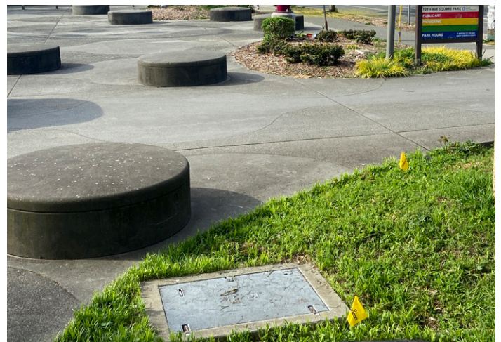
Figure 4.7 Well maintained turf and pavement at 12th Ave Square Park. Photo by author.
