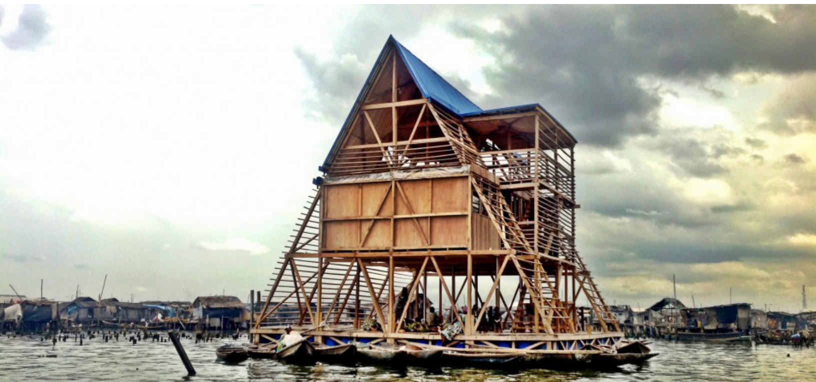
Fig.2.3 Makoko Floating School by Kunle Adeyemi Lagos, Nigeria Source: "Inside Dharavi Slums". http://www.not-home.com/2012/03/inside-slums-of-mumbai.html
