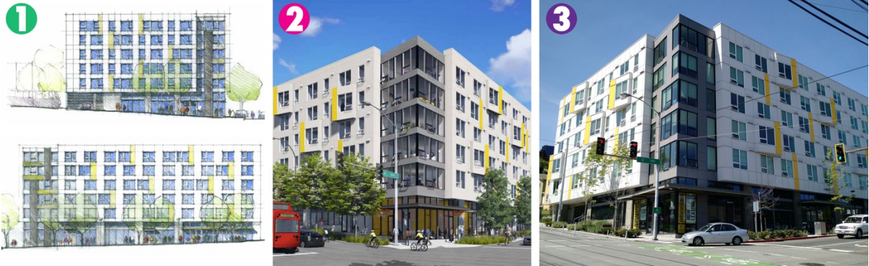
Figure 18: Timeline of design for Anthem. 1) EDG, 2) Recommendation, 3) Final construction. Note the addition of the angled, protruding window bays in the recommendation phase. Sources: EDG and recommendation packets from Mithun, Scott Cutler.
