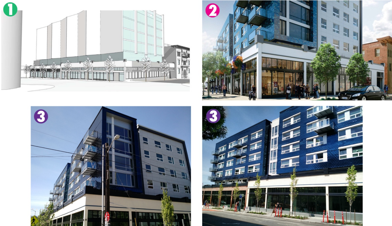
Figure 24: Design timeline for the northern portion of AVA Capitol Hill along E Pike Street. 1) EDG, 2) Recommendation, 3) Final construction from two angles. Sources: EDG and recommendation packets from Ankrom Moisan, Scott Cutler.
