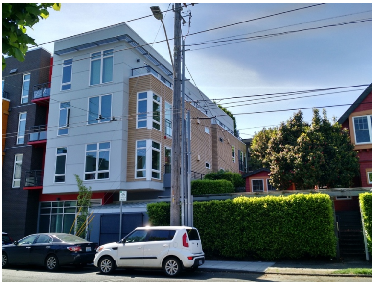
Figure 13: The final setback at the northern transition zone. Note the tiered setbacks as a difference from Figure 11. Source: Scott Cutler.
