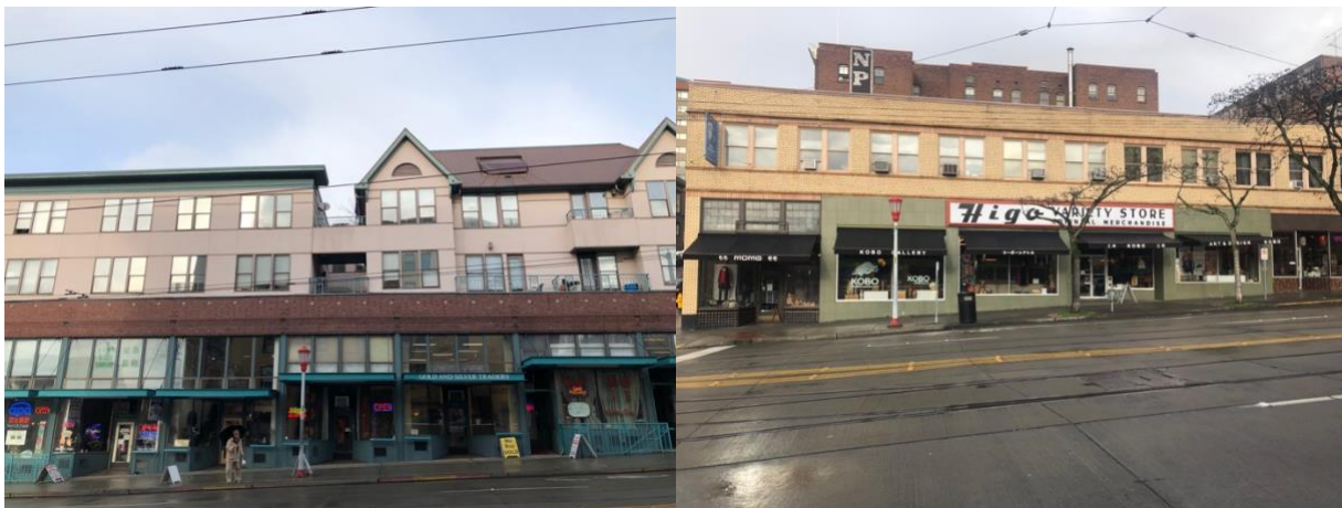
Figure 4-15. Views of C-ID (West of I-5 Freeway)
