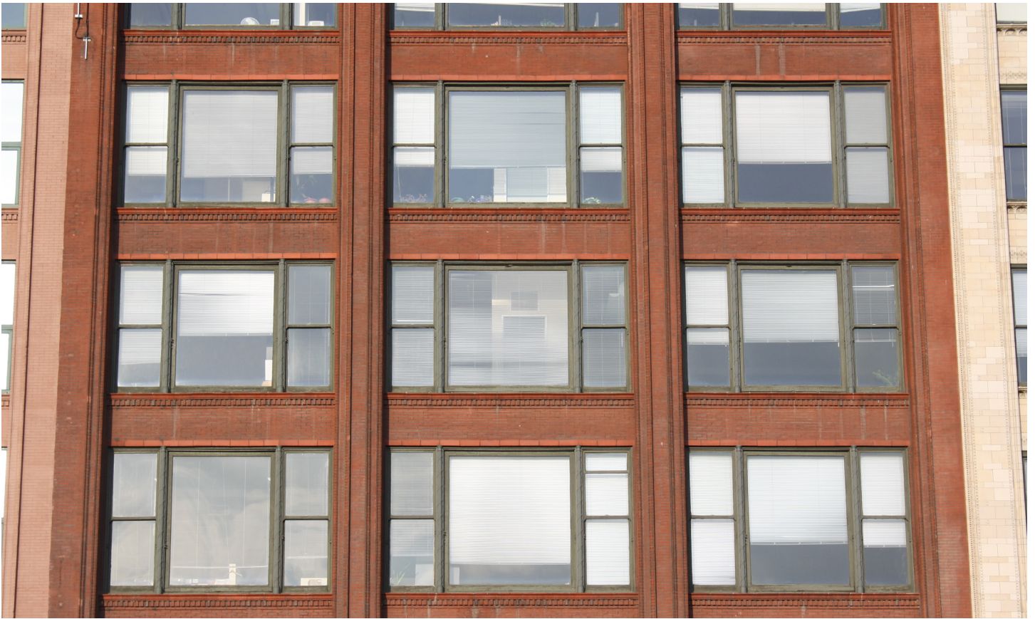
Window mullions can create complexity and order by repeating a similar pattern.
