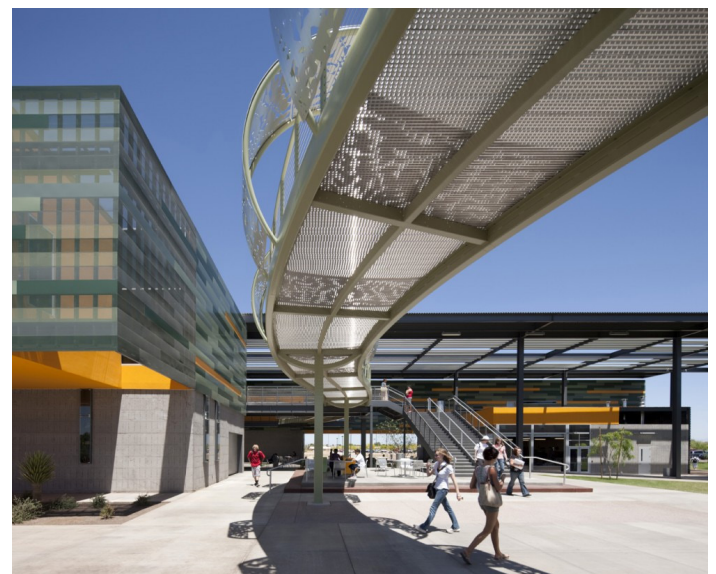
Bridges that lead into the school create a high vantage point for students.
