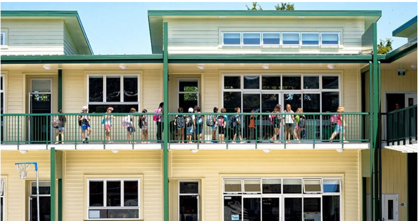
Exterior walkways allow students to view their surroundings while moving between classes.
