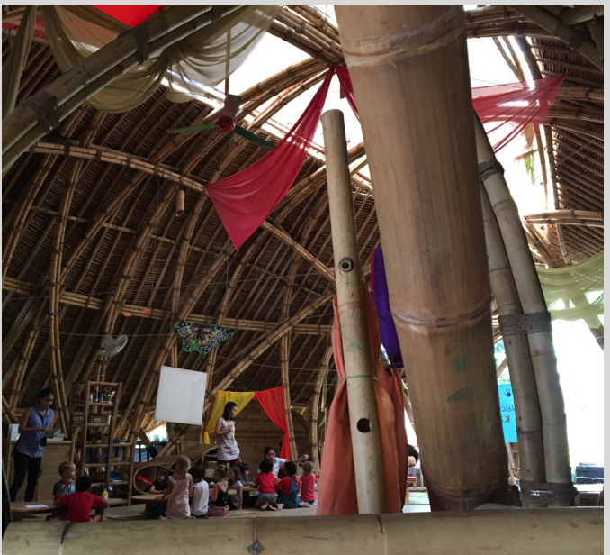
Fig. 2.28. Roof form and skylight of one classroom block
