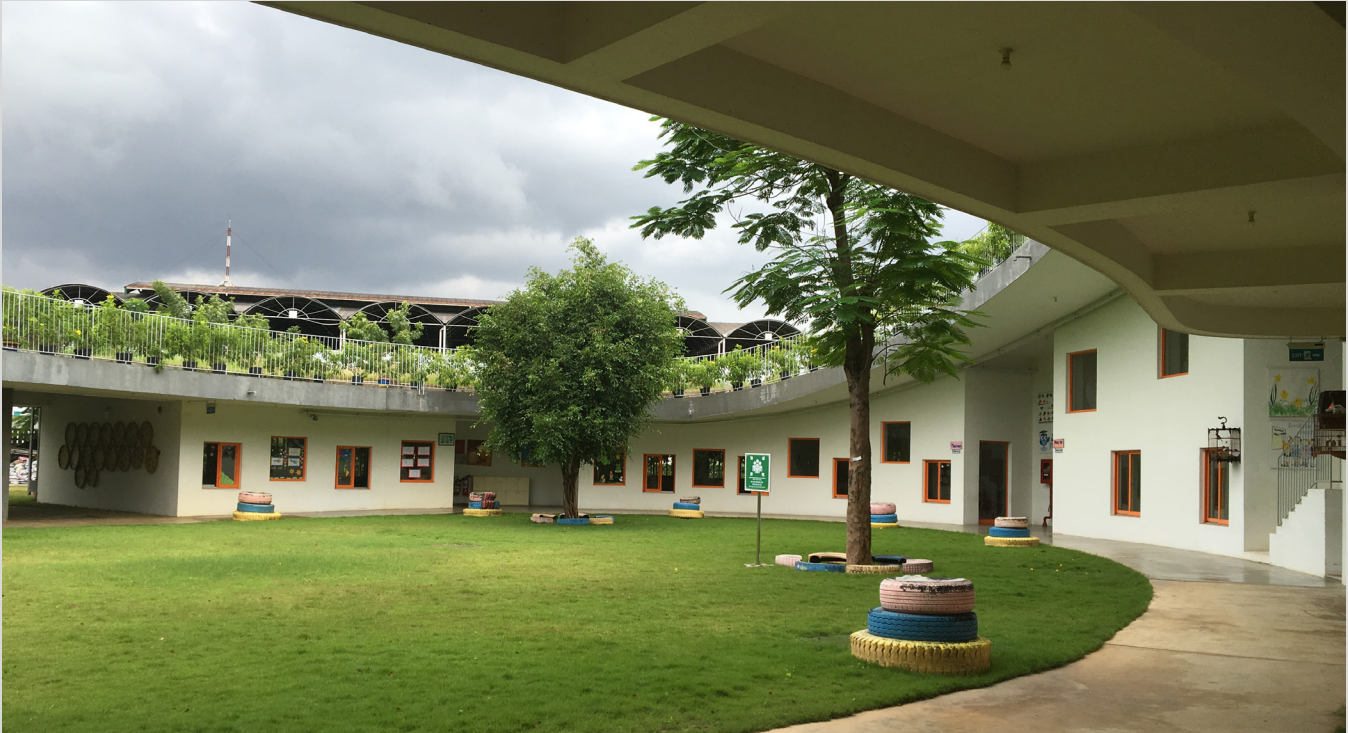
Fig. 2.17. Window configuration of classrooms
