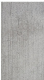
1. Exposed re-inforced concrete framework
