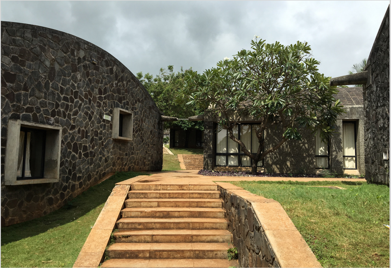
Fig. 2.31. Stairs winding around vaulted boarding school blocks
