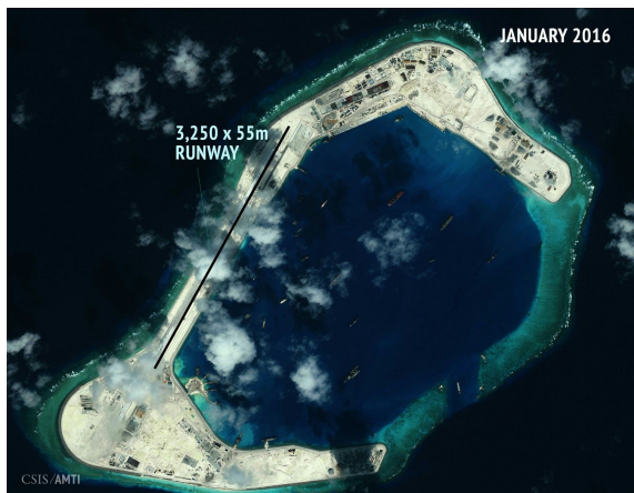
Figure 1.3: Completed airstrip, helipad, buildings, and piers
