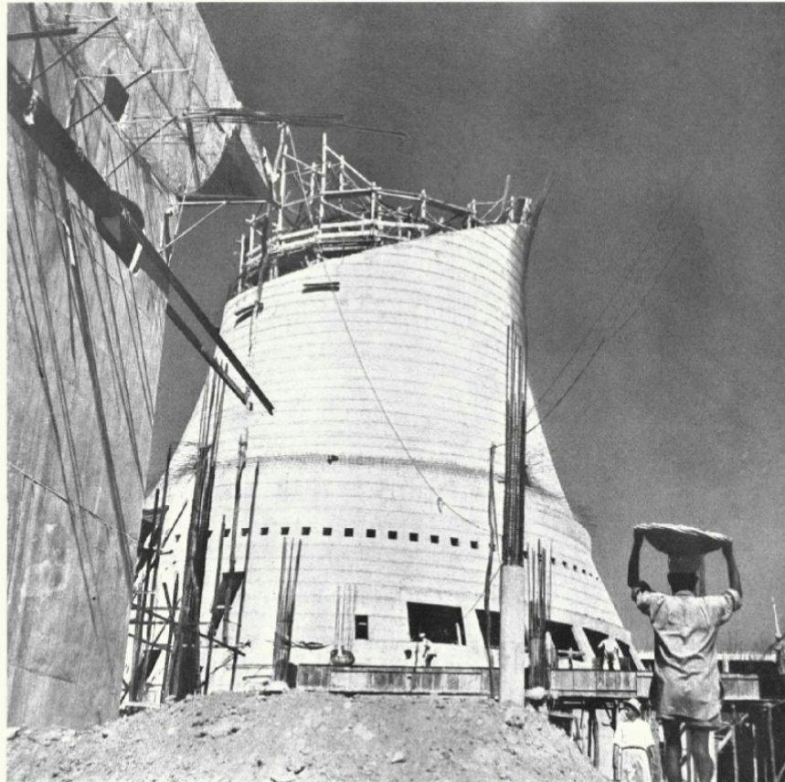
27. The full view of the Assembly Building under construction
