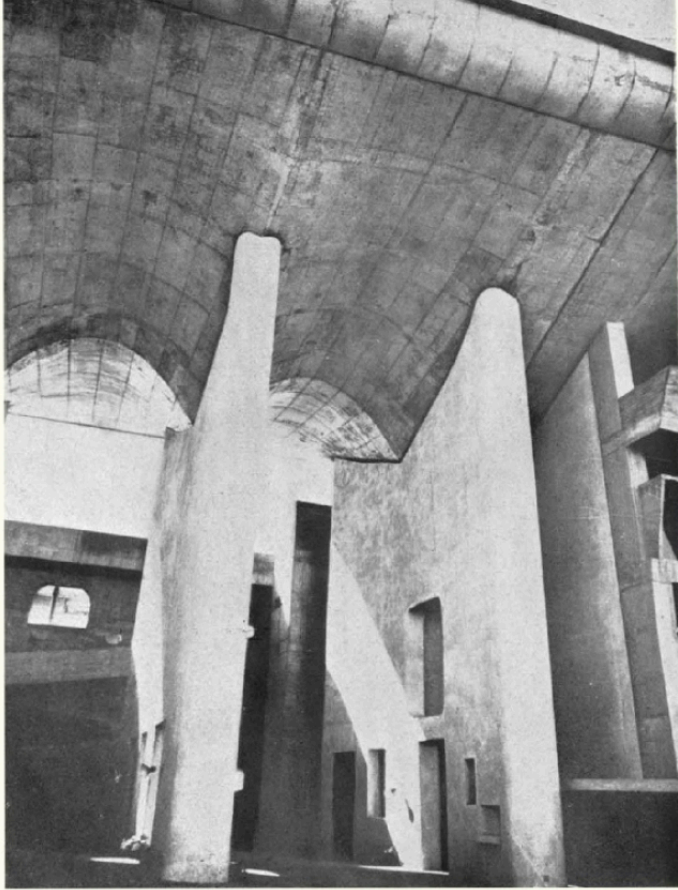
15. Interior of the High Court Portico. Photo by Jeet Malhotra
