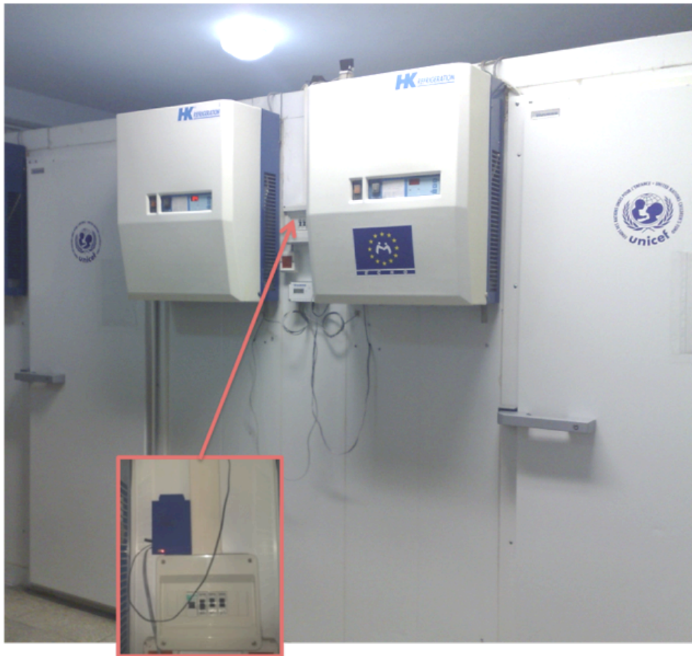
Figure 30: FoneAstra deployed at the country's national store in Tirana, Albania. The FoneAstra box was placed between the two compressors for two cold rooms (note each room's door handles on left and right). Cables from FoneAstra were routed through thermally insulated holes in the walls of the cold rooms and lead to the sensor inside. Photo credit: Ministry of Health, Albania.
