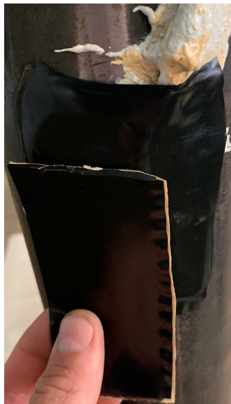
(c) Completed and protected strain gauge
