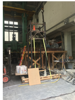
(b) Specimen prepared for base concrete base slab cast
