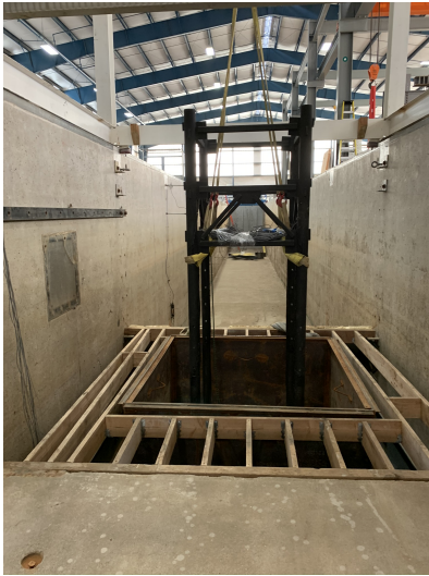
(a) Deck framing under construction
