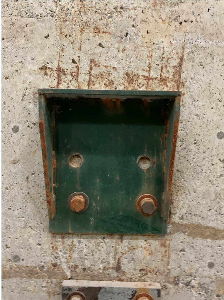
Figure 4.1: Clips bolted to flume wall that concrete slabs rest on
