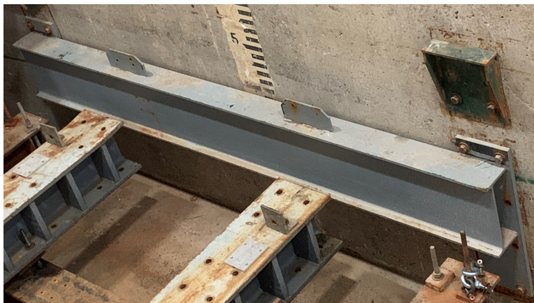
Figure 4.5: Beam attached to side of flume that provides anchorage spots in the middle of the bay
