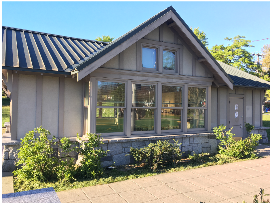
Figure 4.3. Shelterhouse, a renovated amenity in the park.
