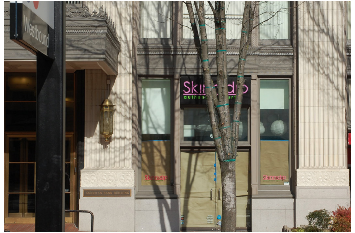
Figure 10 Example of a building that is visible by design only
