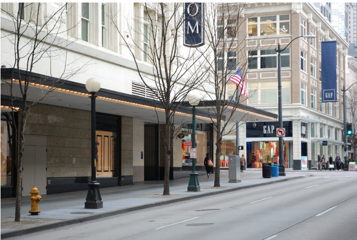
Figure 34 Blank fascades front the streets at the station area.
