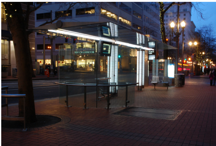
Figure 13 New internally illuminated bus shelter lighting along SW 6th Ave
