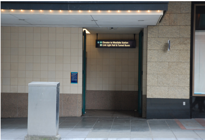
Figure 45 Tunnel entry sign is small and difficult to read.
