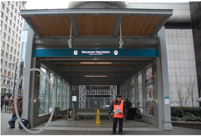
Figure 81 The City Centre Station does not have route information. One possible location for this type of information is circled in the photo above.
