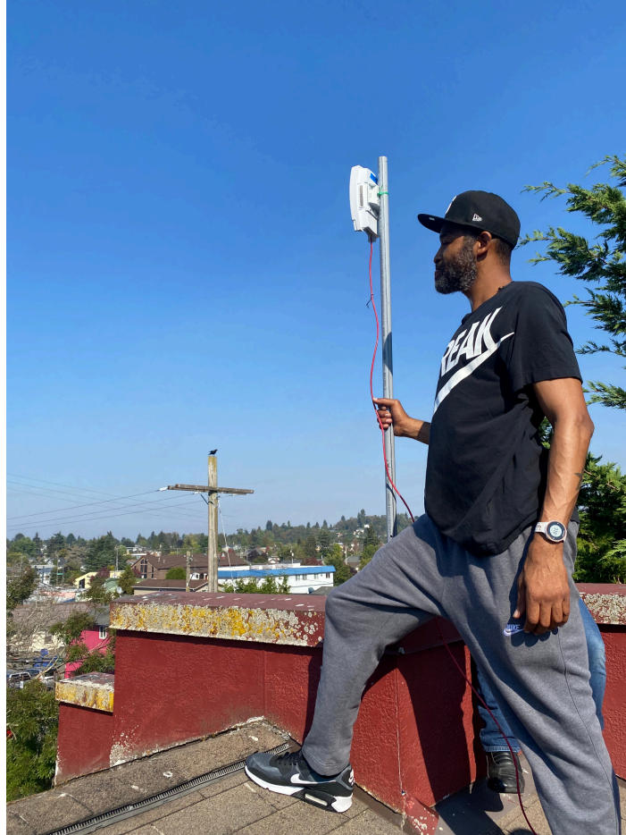
EEC-WA Connect Broadband Technician Performing Site Survey
