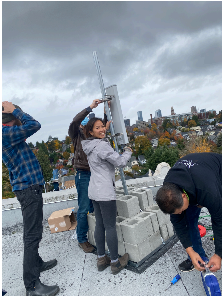
Garfield High School Antenna Mast During Installation
