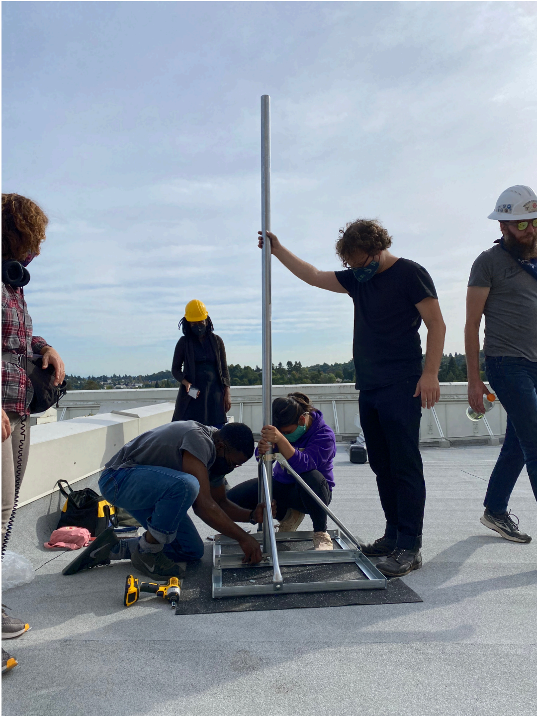
Franklin High School Site Antenna Mast Construction
