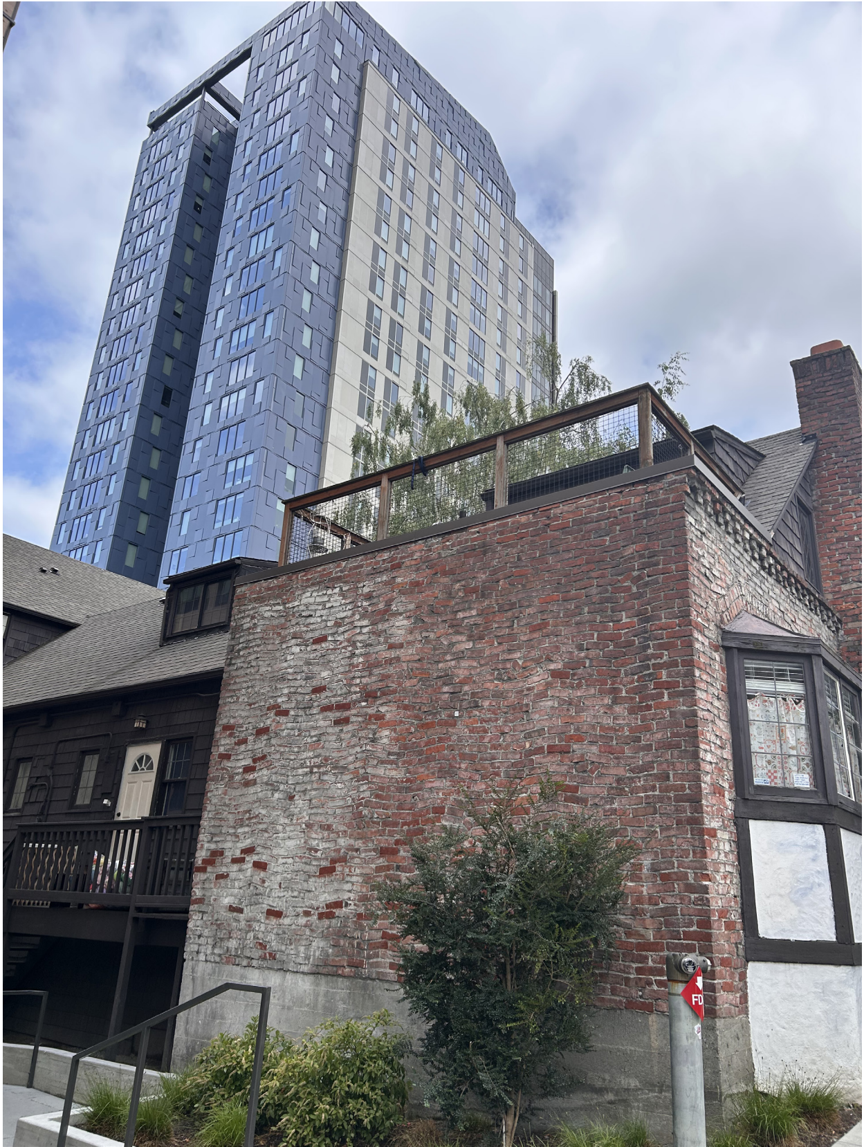
Figure 7. Example of contrasting buildings seen from Brooklyn Avenue NE. Original image by the author.
