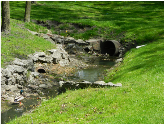
Figure 69 | A current image of the Bloody Run Creek reentering a pipe in Elmwood Cemetery.
