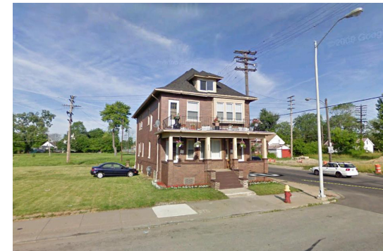
Figure 55| A two-family residential house.
