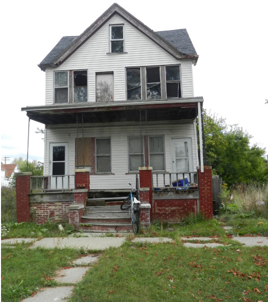
Figure 74 | A typical-style two-family house.
