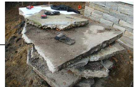
Permeable paving: Broken concrete
