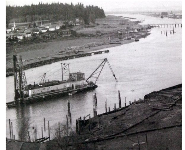
Dredging of the Swinomish Channel, early 1900s.
