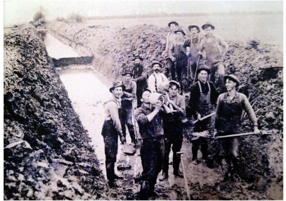
FIGURE 11. DIKE CONSTRUCTION ON THE SKAGIT DELTA
