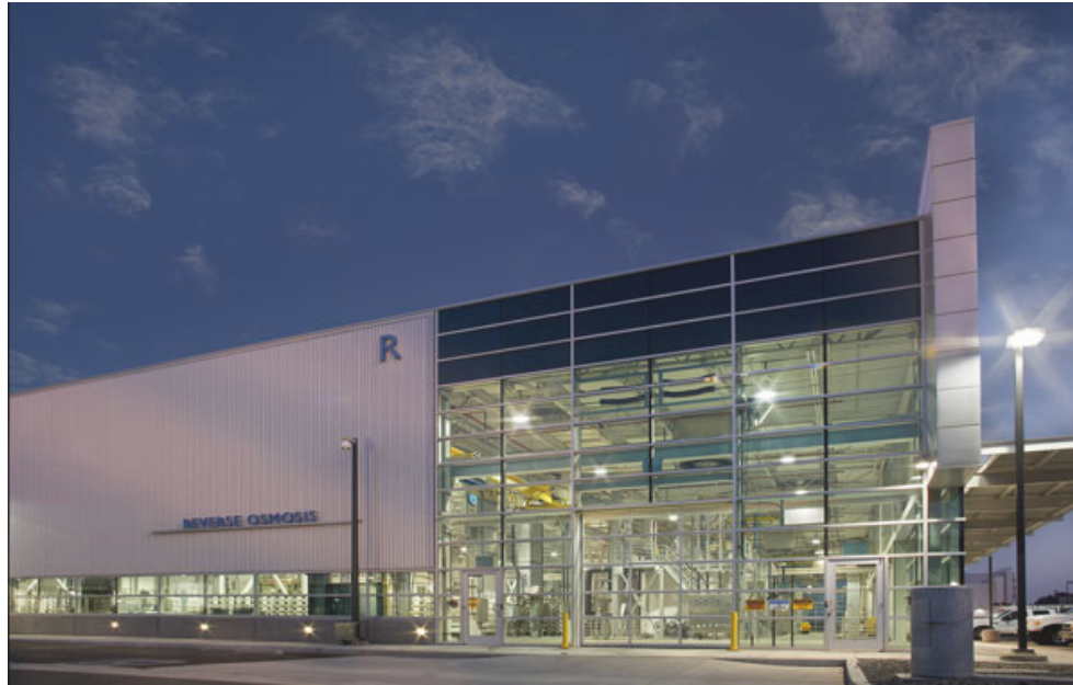
16. The Reverse Osmosis processing building at the GWRS.
