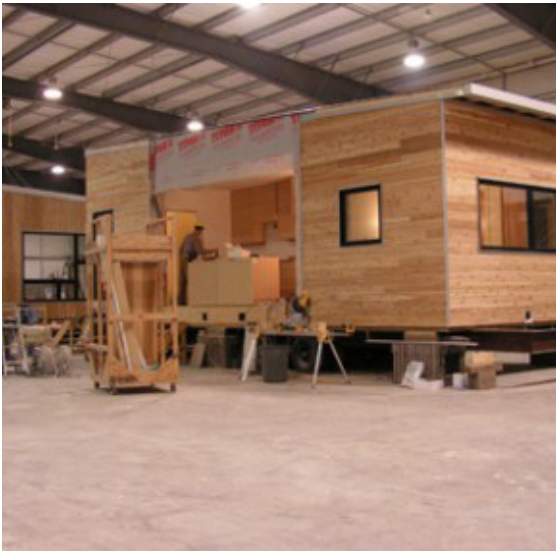
Figure 79: Prefabricated Construction in a factory controlled environment.
