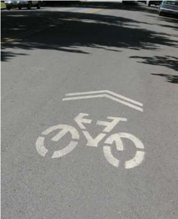
(e) A shared-lane marking, commonly known as a sharrow, located on a street open to all traffic. Photo by NACTO, location unknown.
