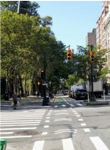
(c) A higher quality, moderately expensive parking-protected bike lane with dedicated signals. Photo by author, New York City, NY
