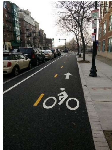
(d) An expensive but top quality, parking-protected and grade separated cycle track with dedicated signals. Photo by author, Boston, MA
