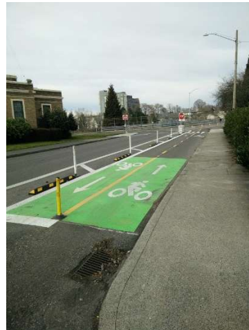
(b) A higher quality yet still inexpensive quick-build separated bike lane. Photo by author, Portland, OR
