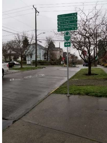
(f) A higher quality neighborhood greenway with wayfinding signage and physical traffic calming that permits all users. Photo by author, Seattle, WA
