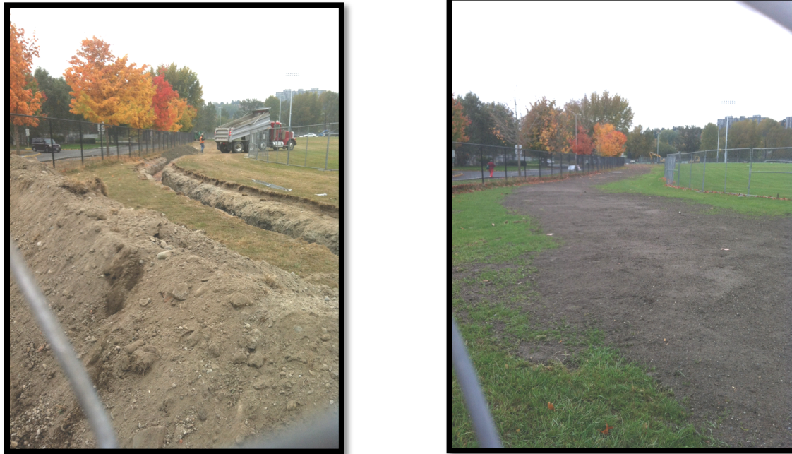
Figure 2: Soil disturbed during construction of an irrigation pipe for the Intramural Fields at the University of Washington. Soil was mechanically excavated one day and stockpiled during the pipe construction (photo on left). The soil was then replaced two days later (photo on right). The area was then hydro-seeded making the large amount of soil excavation and replacement almost invisible.
