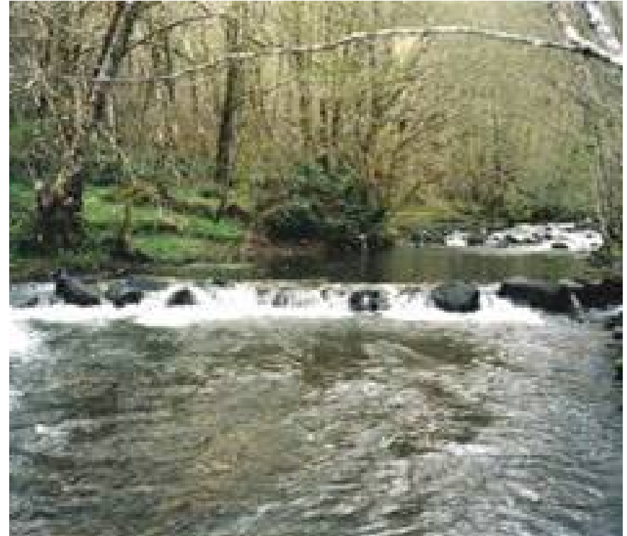
Log weirs placed in a small coastal Washington stream to create pools and habitat for coho salmon. NWFSC.
