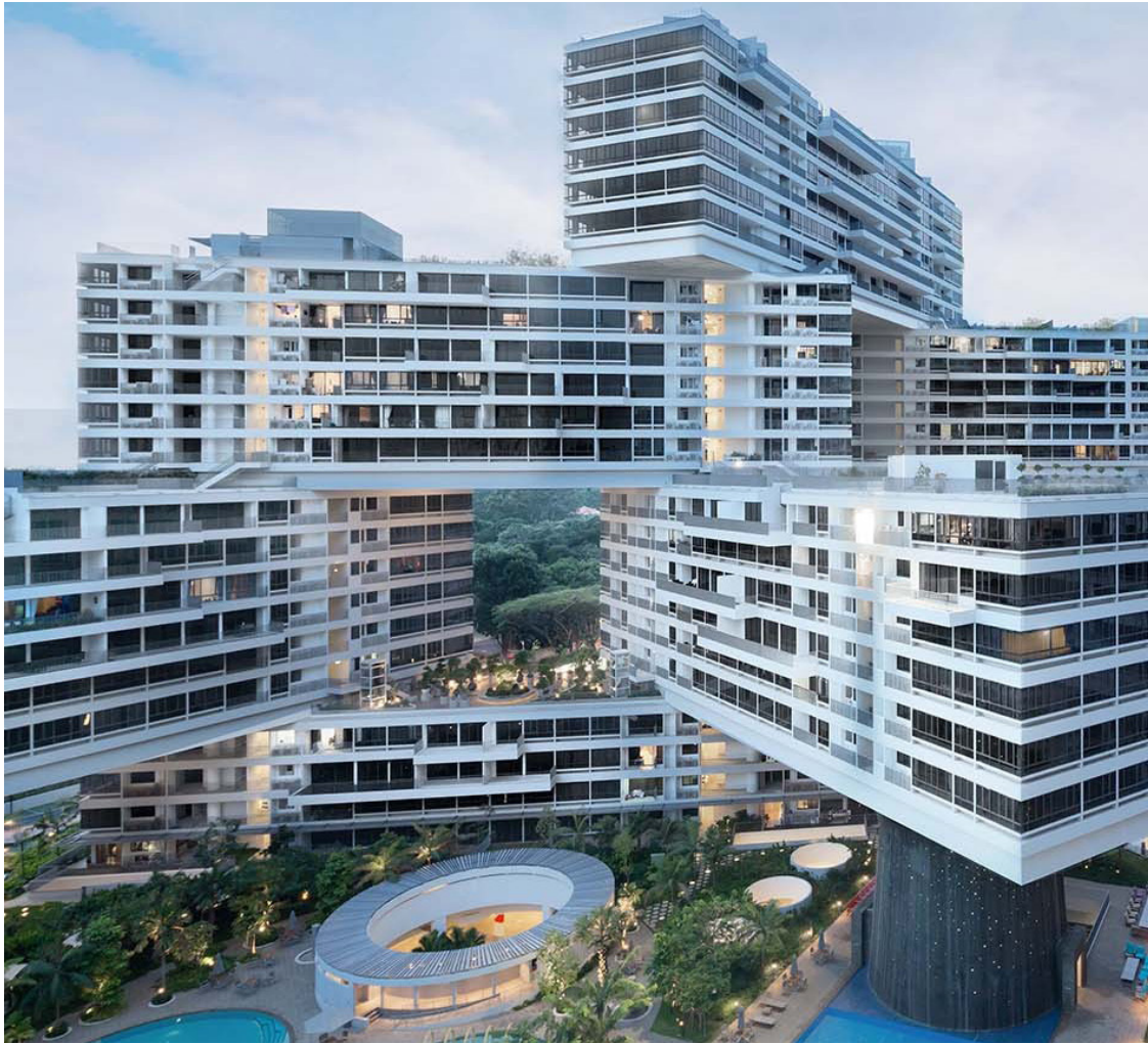
Figure 20: Though uniform in massing, the stacked blocks create a varied vertical experience and open the ground plane up for landscape and amenity space.
