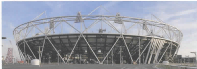
"The steel columns... have bolted connections rather than connections welded on site.
