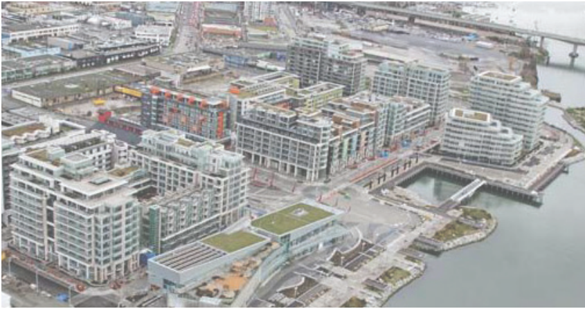
Figure 22: The Olympic village at False Creek, part of Vancouver's 2010 Olympic development failed to find residents immediately after the games due to poor construction, non-competitive pricing, and a typology not analogous with the rest of Vancouver. and provide no real positive impact on the city?
