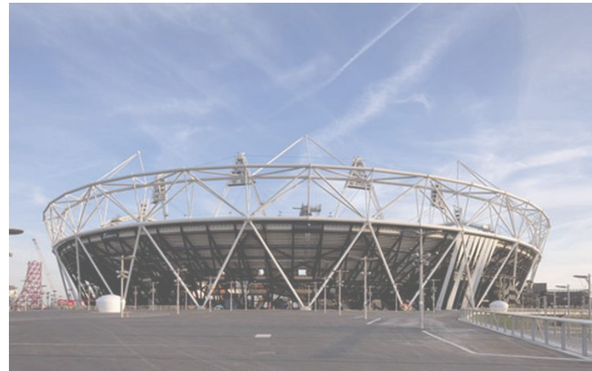
Figure 25: Populous's main stadium has been transformed into an arena for the West Ham soccer team - a costly construction process but one that keeps the site in use. Instead of the original 80,000 spectators, it can now hold 64,000.
