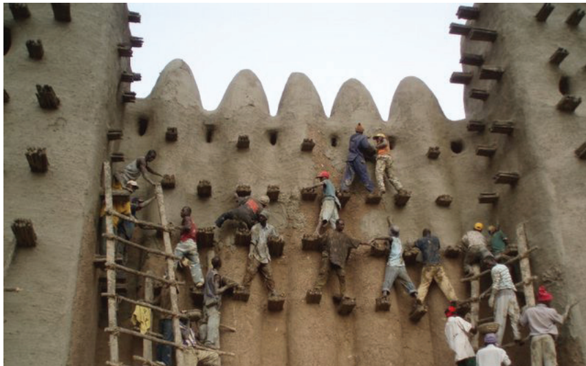
Figure 5: In anticipation of the rainy season, the mud-plaster on the exterior of the mosque must be replaced. This is increasingly important with the onset of climate changes that have increased desertification of the region.
