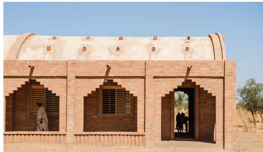
Figure 6: The primary school designed by LEVS pushes mud-brick construction to be a more advanced construction method. However, this roof was not original, but retrofit as an accommodation to UNESCO's requirements for material expressions to be consistent with the Dogon design principles.
