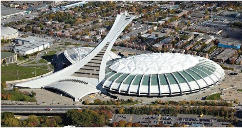
Figure 19: Tallibert's stadium in Montreal. The roof is meant to be retract but has failed many times in the past.
