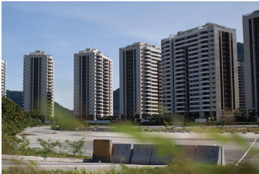
Figure 29: The athlete's housing, hastily developed, is relatively unoccupied. In order to build the stadiums, an existing neighborhood of nearly 70,000 Brazilians was evicted from their favelas.
