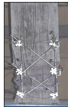
Figure 3.5 (F8) Longitudinal Bar Fracture
