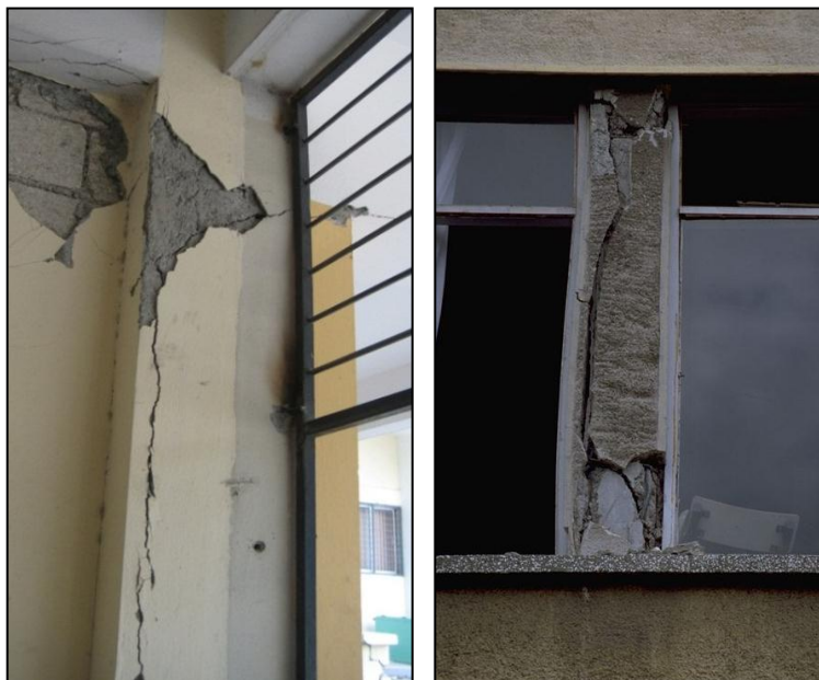
Figures 3.76 (Sedra, et al. 2010) and 3.77 (PEER) Longitudinal cracking on side faces: earthquake damage
