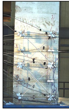
Figure 3.16 (F1 & F2) Flexural and Longitudinal Cracking
