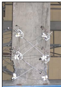
Figure 3.9 (F6 & F7) Longitudinal Bar Buckling and Crushing of Core Concrete
