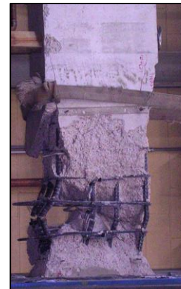
Figure 3.21 (F8) Longitudinal Bar Fracture
