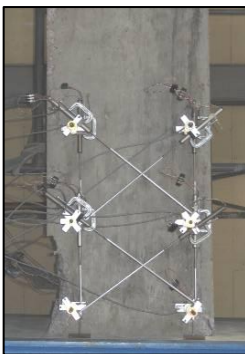
Figure 3.7 (F4) Concrete Spalling on Flexural and Side Faces
