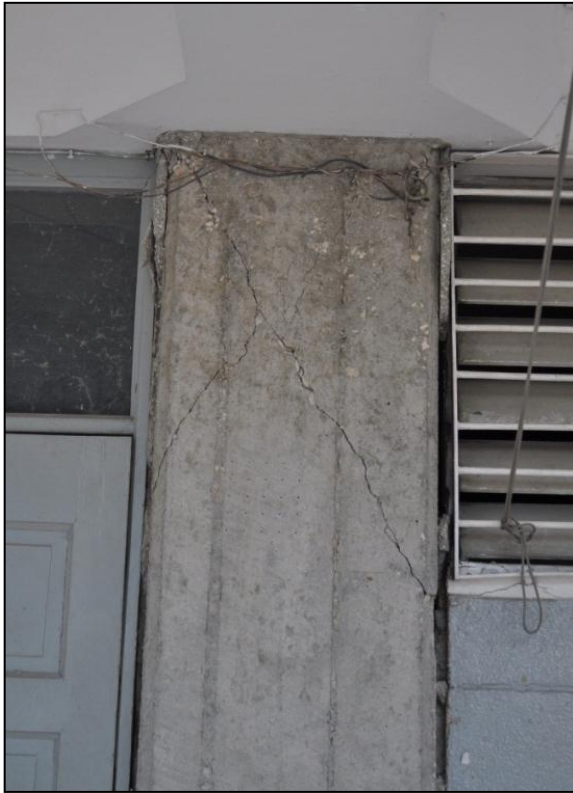
Figures 3.63 and 3.64 Shear cracking on side faces: earthquake damage (Sedra, et al. 2010)
