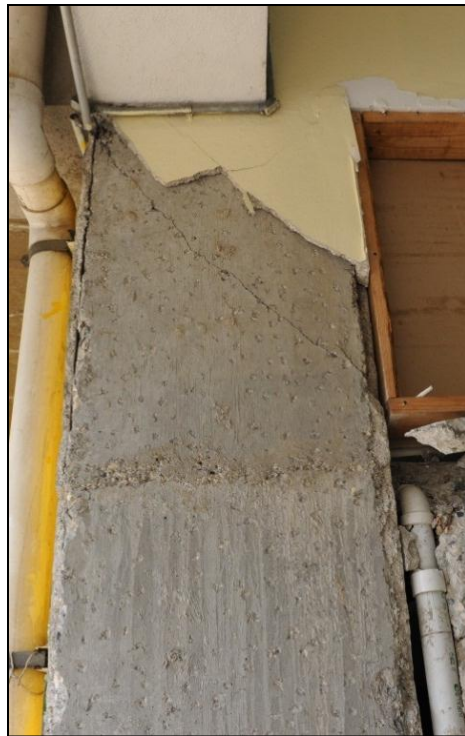
Figures 3.65 and 3.66 Shear cracking on side faces: earthquake damage (Eberhard, et al. 2010)
