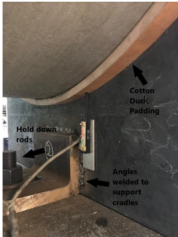
Figure 3-21. Support cradle arrangement
