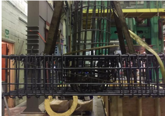
Figure 6-11. Reinforcement cage for cap beam being lifted into formwork for casting
