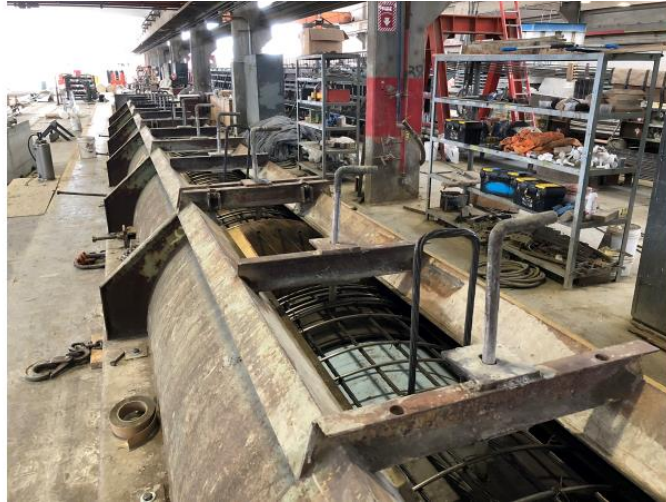
Figure 3-10. Pile-column formwork ready to be line-cast at Concrete Technology Corporation
