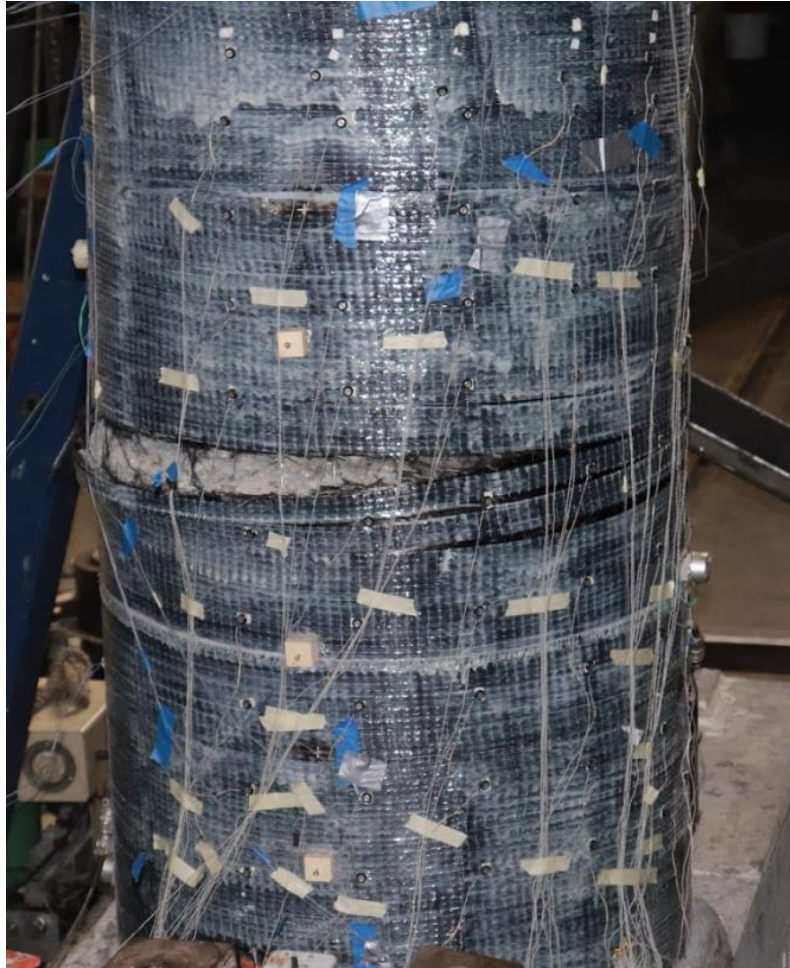
Figure 7-14. Fiber rupture on north face during Series 11
