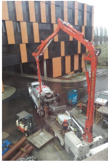
Figure 3-13. Concrete pump truck used for fill concrete
