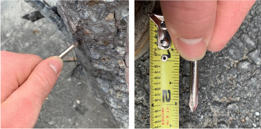
Figure 7-23. Measuring of the strand slip
