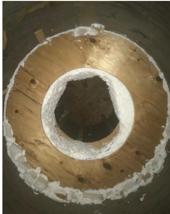
Figure 3-15. Foam spacer followed by last plywood ring
