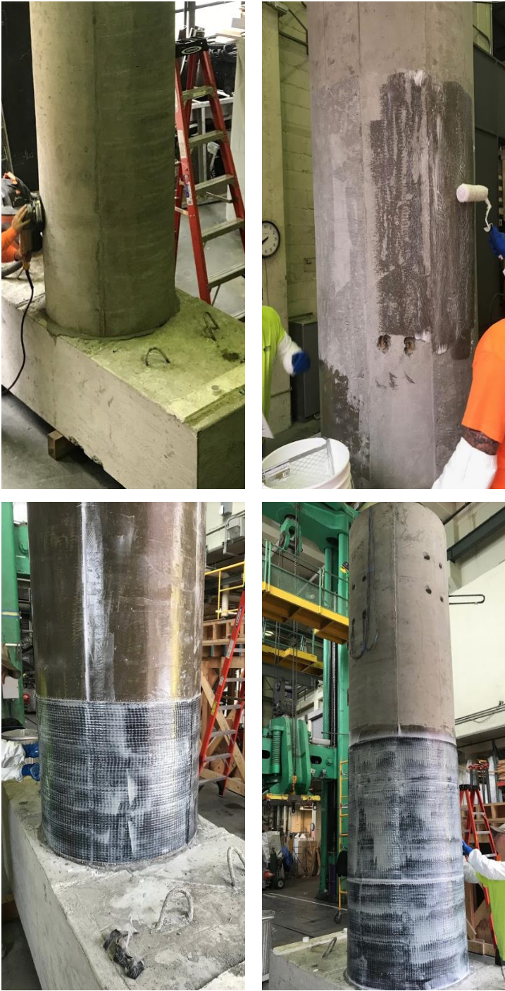
Figure 6-17. CFRP application: sanding concrete (top left), base epoxy (top right), first layer of CFRP (bottom left), finished epoxy (bottom right)
