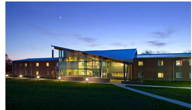
Figure 8 - Potomac Job Corps exterior. Credit: CGS Architects.
