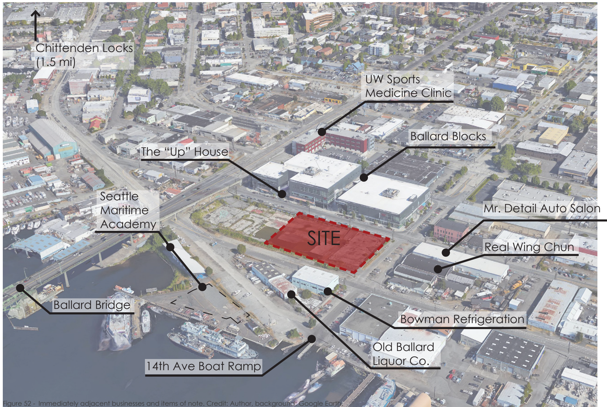
Figure 52 - Immediately adjacent businesses and items of note. Credit: Author, background: Google Earth.
