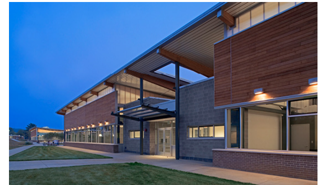
Figure 7 - Potomac Job Corps exterior. Credit: CGS Architects
