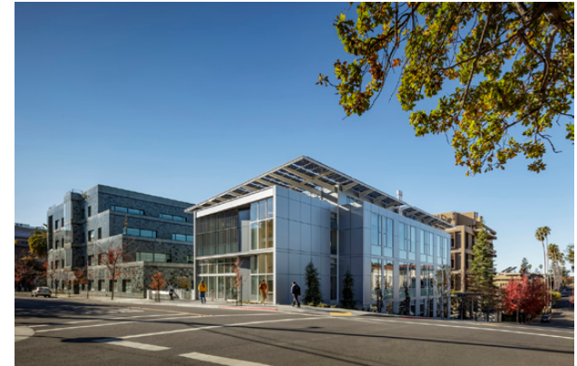
Figure 34 - Exterior. Credit: Tim Griffith.
