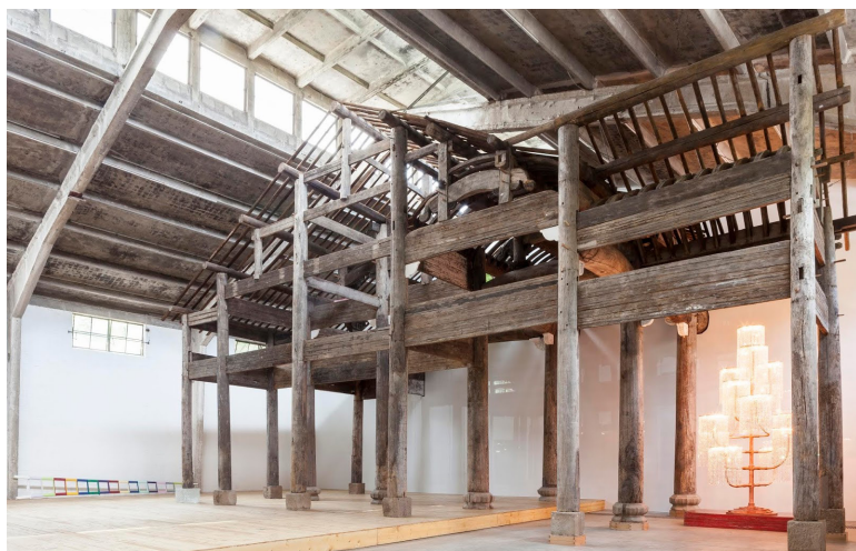
Figure 47. Wood frame structure of Hui Zhou architecture
