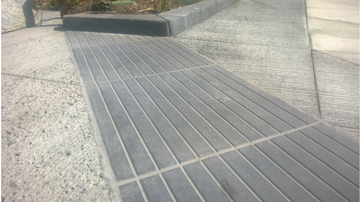
Figure 6. Textured paving informs visually impaired users that they are approaching the travel way
