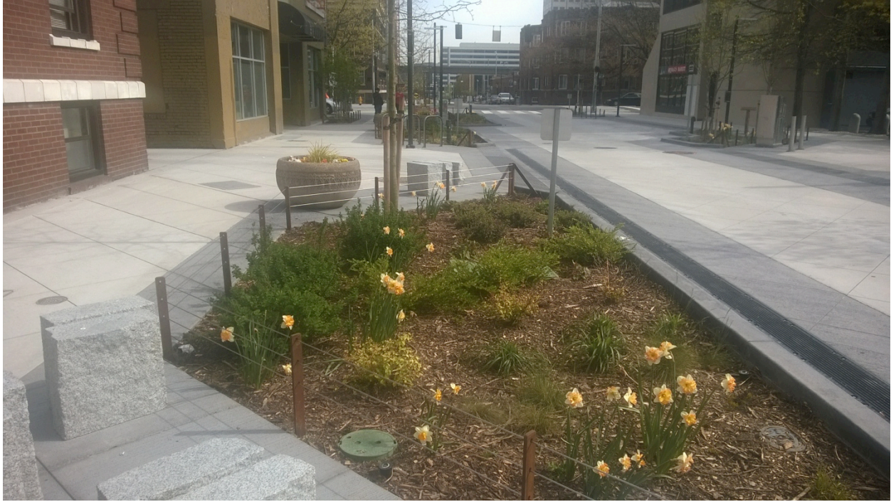
Figure 7. Rain gardens capture storm runoff and provide a buffer between the sidewalk and travel way
