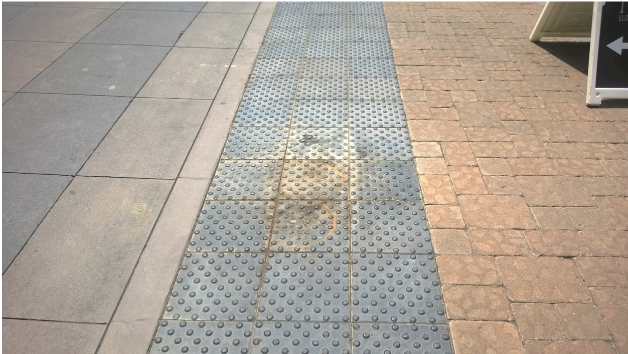
Figure 29. Tactile warning strips separate the at-grade roadway from the adjacent sidewalk
