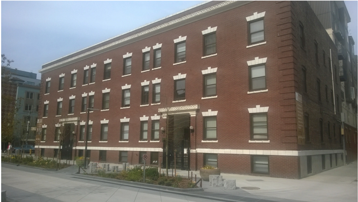
Figure 11. Mid-rise apartment buildings are common along the Bell Street Park
