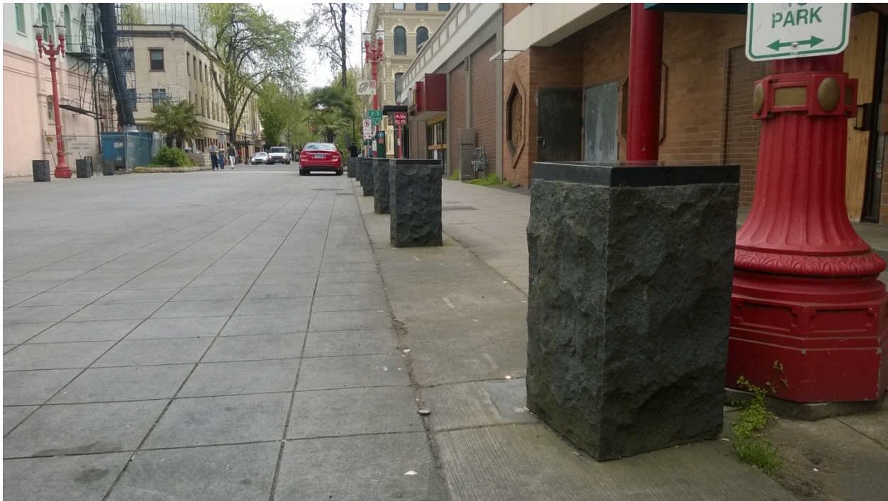
Figure 19. Curbless sidewalks are instead lined with granite bollards
