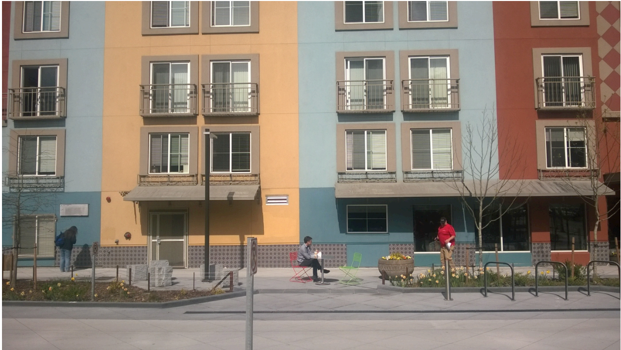
Figure 12. Typical on-street activity along the Bell Street Park
