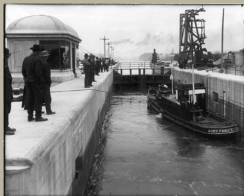
Ballard locks under construction, 1916
