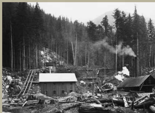
Skagit Dam construction site, 1921
