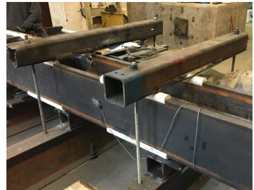
Figure 3.16: Installed out-of-plane restraints.
