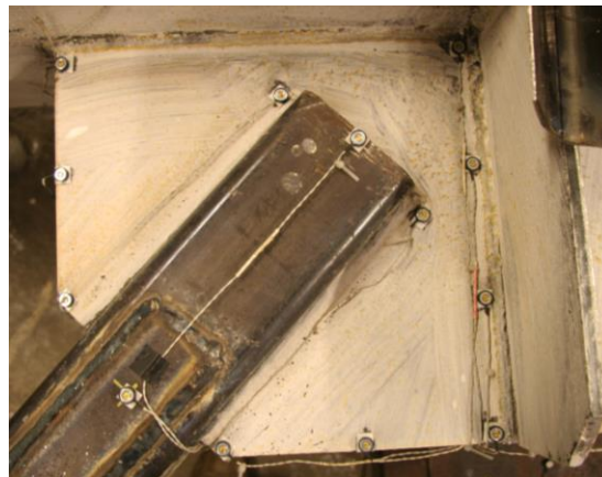
Figure 3.30: Optotrak LEDs on midspan gusset.
