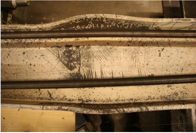
Figure 4.82: S col. severe local buckling at -3.3% drift (LB3-OF).
