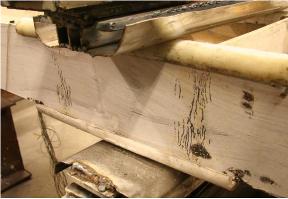
Figure 4.65: Beam yielding at 0.83% drift (Y1-OF).
