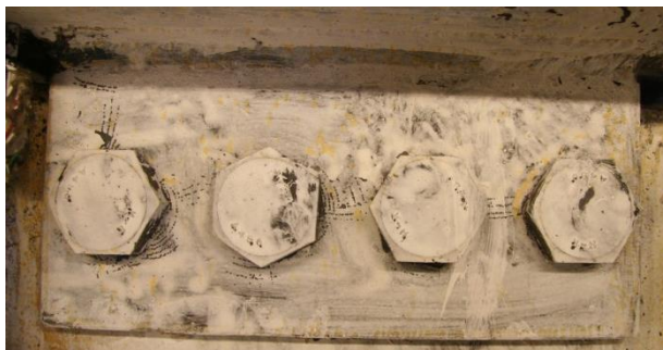
Figure 4.35: Shear tab yielding at 0.83% drift (Y1).
