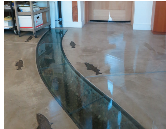
Figure 2.48 A “stream” running through the Science Wing brings rainwater off the roof before being treated, making the hydrological cycle a design element and visible to the students.
