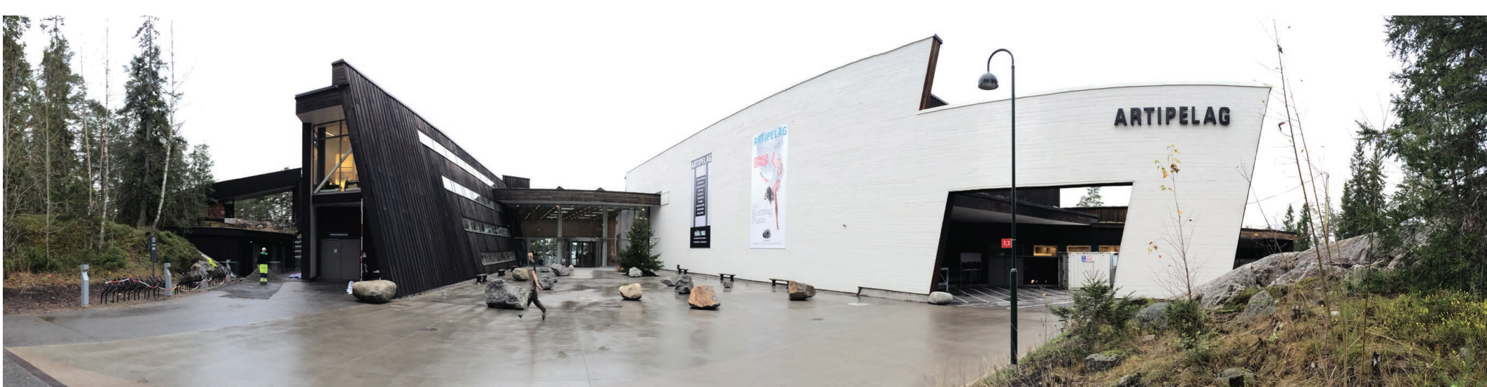
Figure 3.25 Artipelag. Entry court from land
