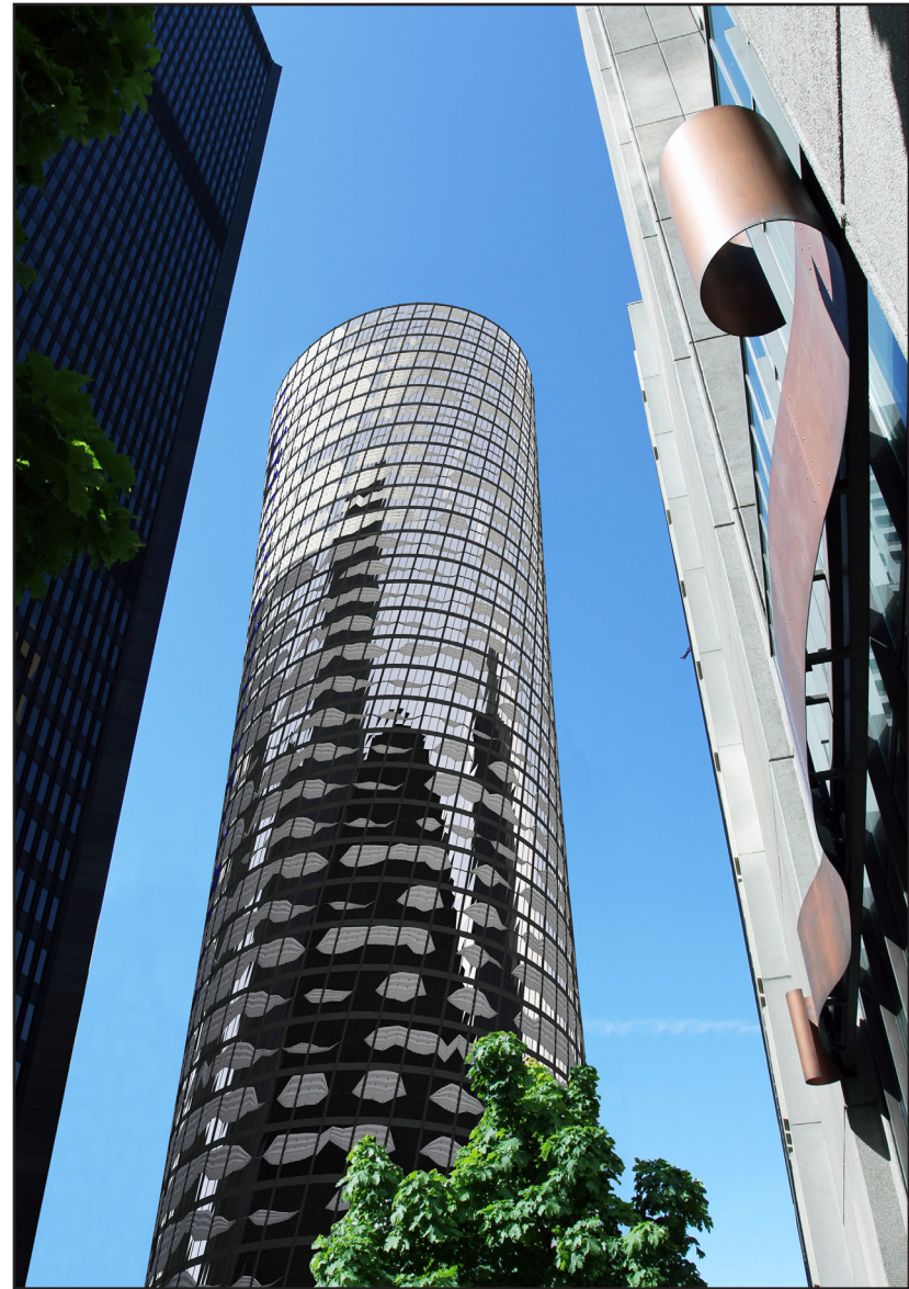
Figure 5-23: Northwest View, ShadeFan system applied on the building facade at the project site
