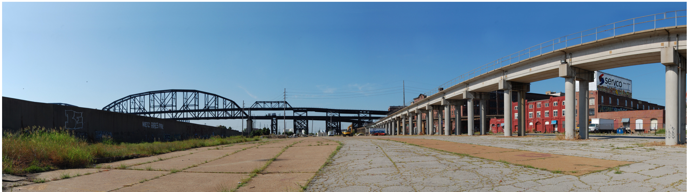
45. View of the project site from the north.
