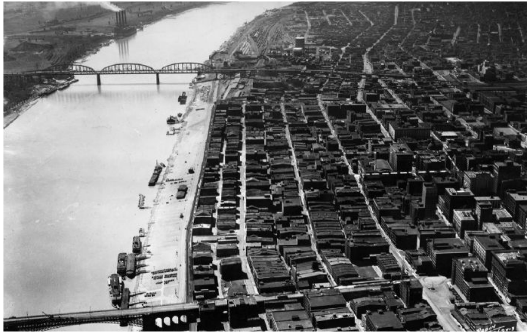
16. The riverfront before clearance for the Jefferson National Expansion Memorial.
