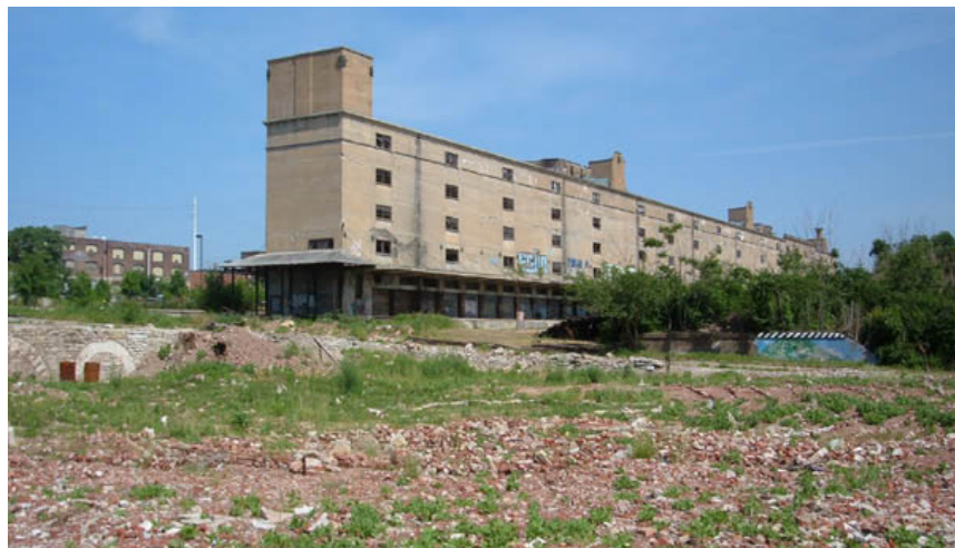
31. The Southwestern Rail Freight Depot.
