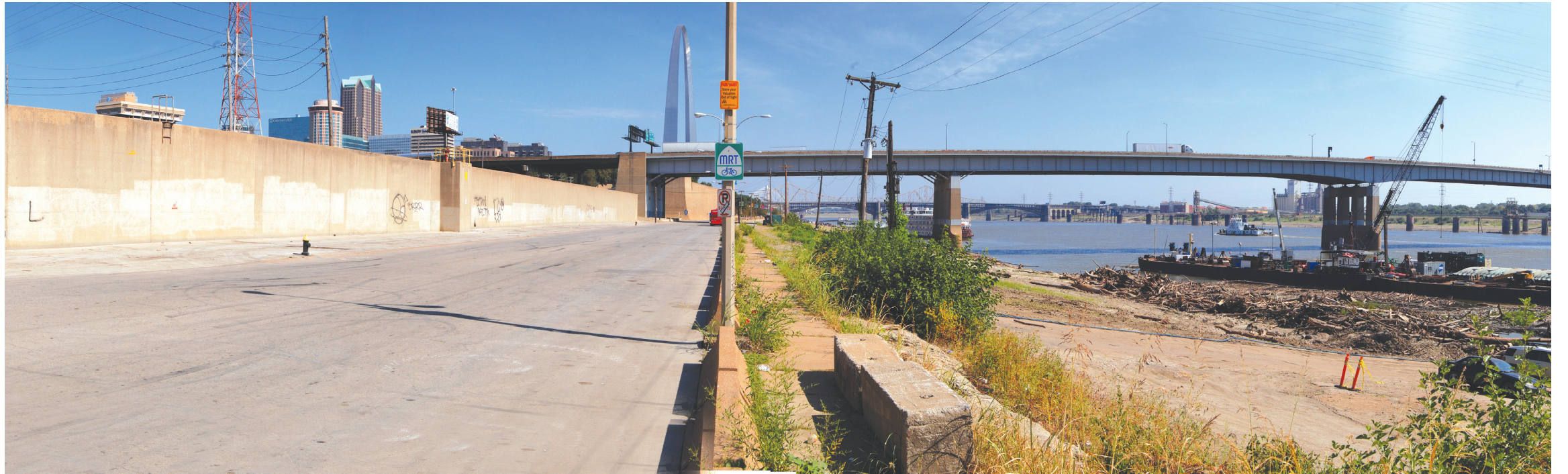
46. The the river side of the flood wall bordering the site.
