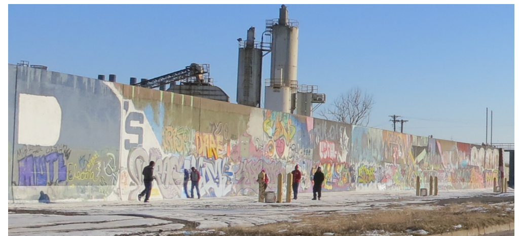
20. Examples of the highways, rail lines, and flood wall.
