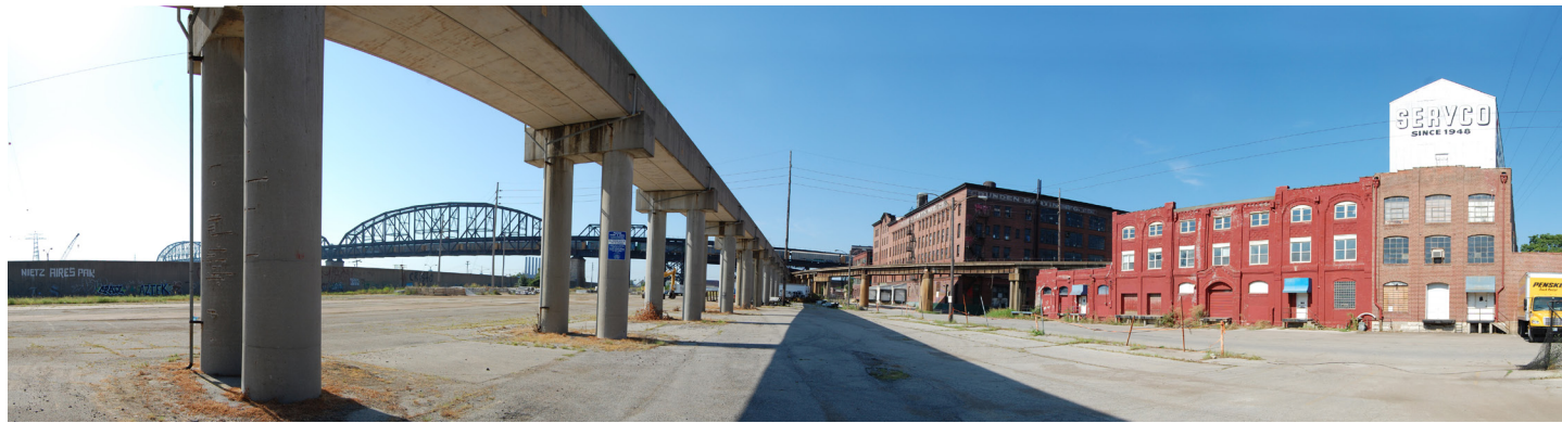
41. Elevated railway bordering the site to the west.
