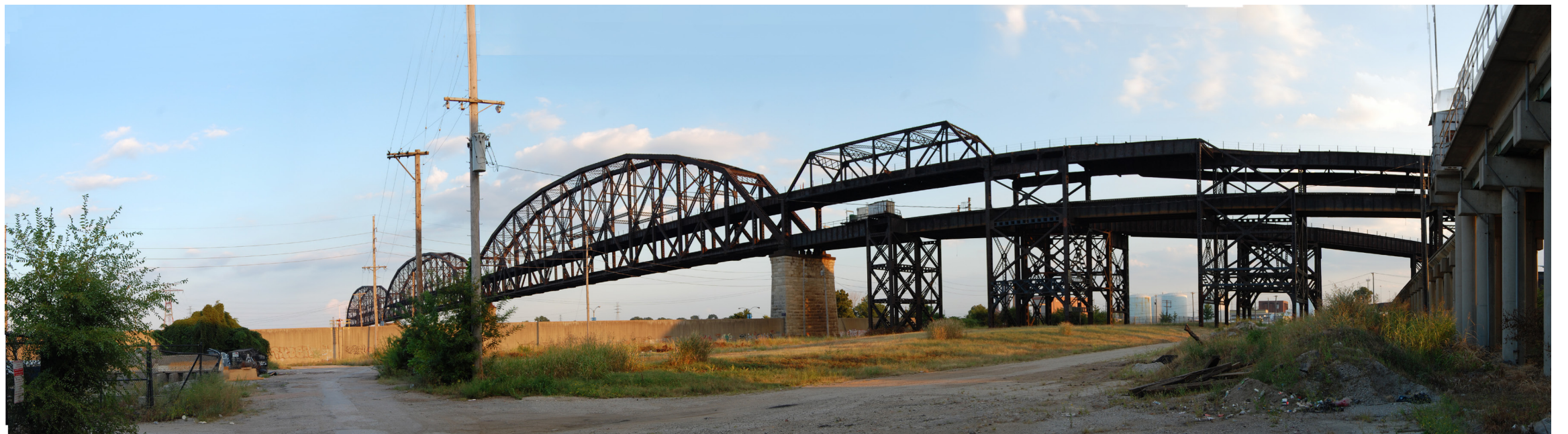
47. The MacArthur Bridge bordering the site to the south.
