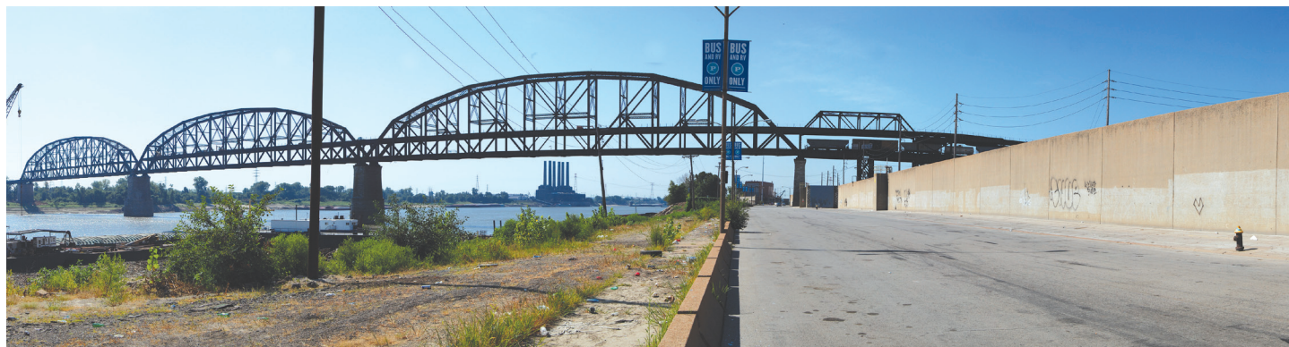
43. Looking south along the flood wall towards the MacArthur Bridge.
