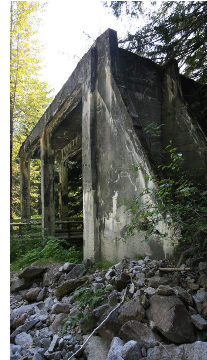
13. Concrete shed cutting into the hillside
