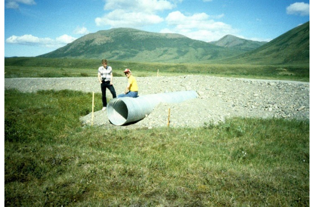
Figure 7-11 A culvert with an extended outlet
