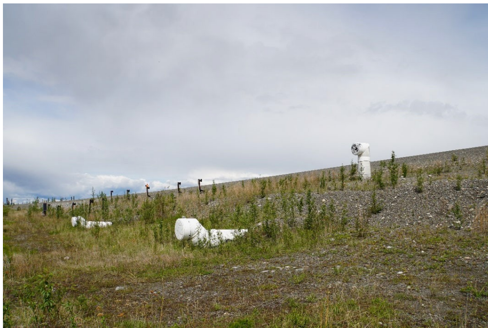
Figure 5-8 Air Convection Culverts with Chimney (Zarling, 1984)
