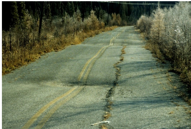
Figure 7-8 Thawing of deep ice wedges on the abandoned section of the Richardson Highway east of Fairbanks
