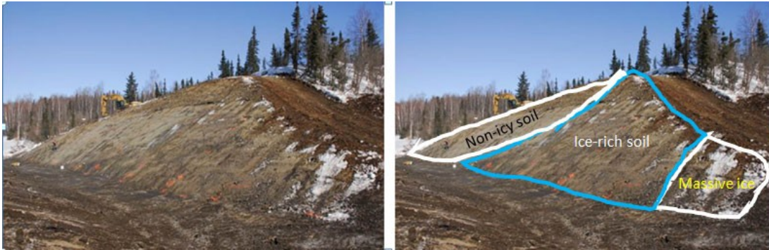
Figure 6-1 Three material types exposed in a permafrost cut slope, before any thaw.
