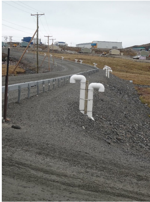
Figure 5-11 Heat drains in Salluit, Nunavik, Canada (photo B. Connor)
