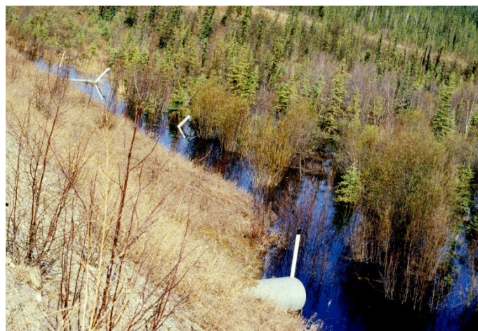
Figure 7-5 Water ponding in a talik formed at the toe of the slope.
