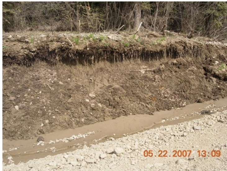
Figure 6-4 Advanced cut slope thaw with silty runoff flowing in a ditch and general slumping of coarse material.
