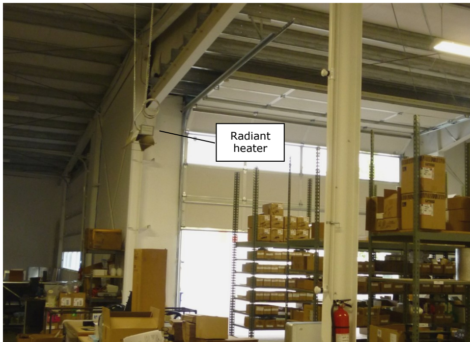
Figure 7 - Interior photo (4) of E warehouse, after to occupancy
