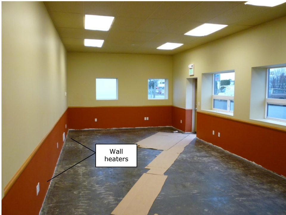
Figure 5 - Interior photo (2) of the office, prior to occupancy
