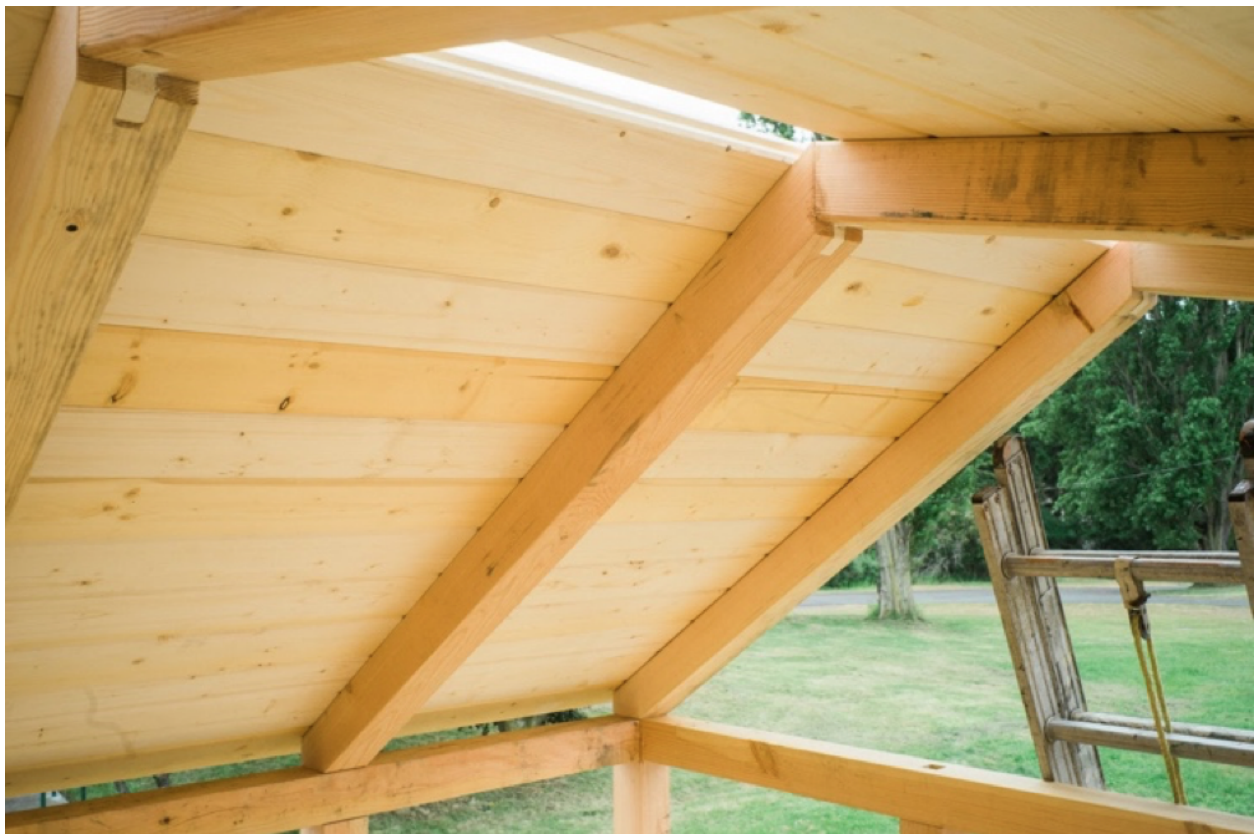
Figure 4: Roofing joinery takes the grain's movement into account, while the small, lighter colored splines in the uppermost joints make for visually interesting wear as the grain moves, gaps, and ages.
