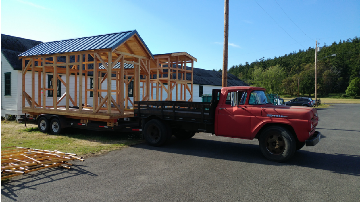
Figure 1: Completed timber framed structures being moved to their semi-permanent sites
