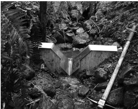
Weir and stilling well (pressure transducer inside) installed at Capitol Forest.
