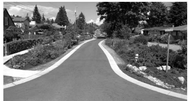
An example of Street Edge Alternative (SEA Street) Project.
